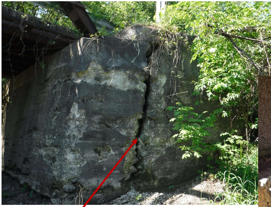
Wide vertical crack in northwest wingwall. Crack expected to be full depth.
