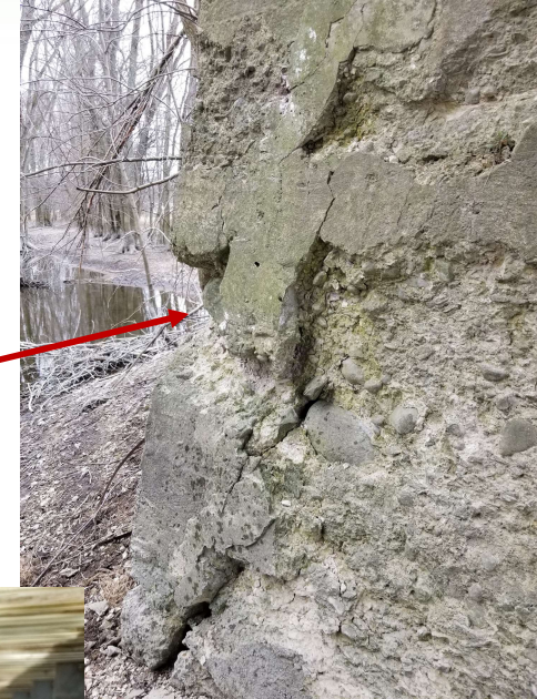
Large vertical crack and spalling at south corner of west abutment.
