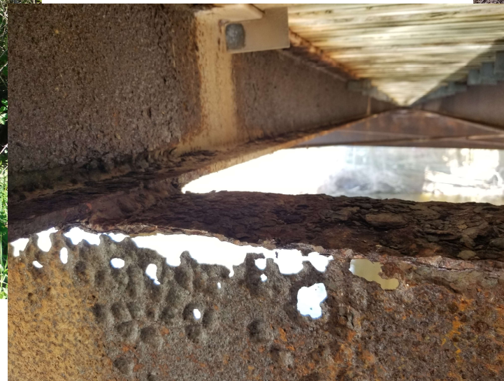
Large perforation at top of cross-beam resulting in significant section loss.
