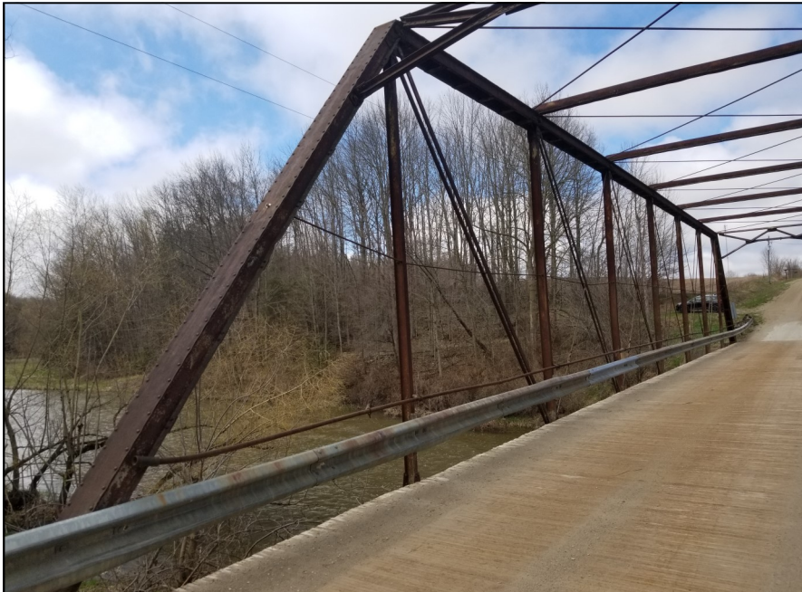
Photo 2 - View of south truss (May 1, 2020)
