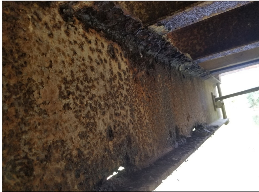
Photo 11 - Severe corrosion, section loss and perforations at east cross beam (September 22, 2020).
