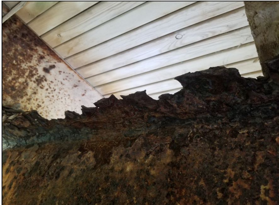
Photo 12 - Approximately 80% section loss at top flange of cross beam (September 22, 2020).
