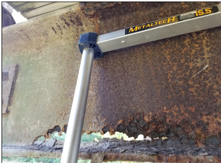
Photo 14 - Large perforation (350mm x 50mm) at north end of cross beam near mid span (September 22, 2020).
