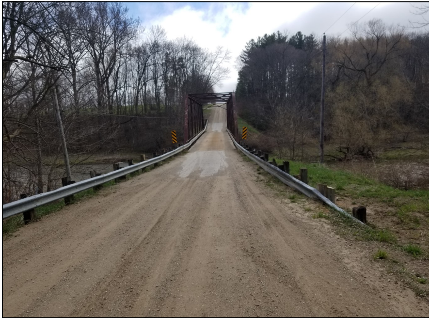
Photo 1 - View of structure from west (May 1, 2020).
