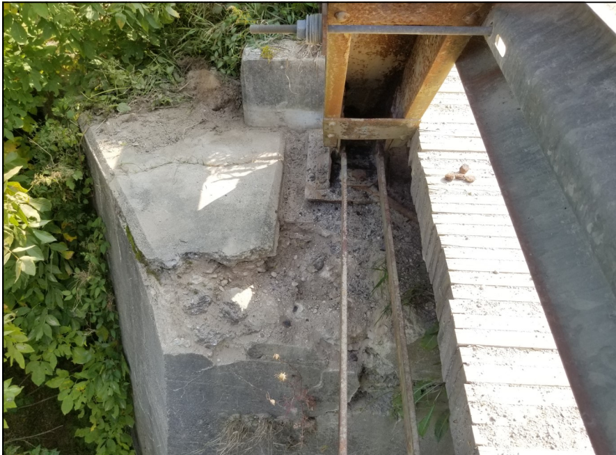
Photo 16 - Significant concrete deterioration and spalling noted adjacent to northeast bearing connection (September 22, 2020).
