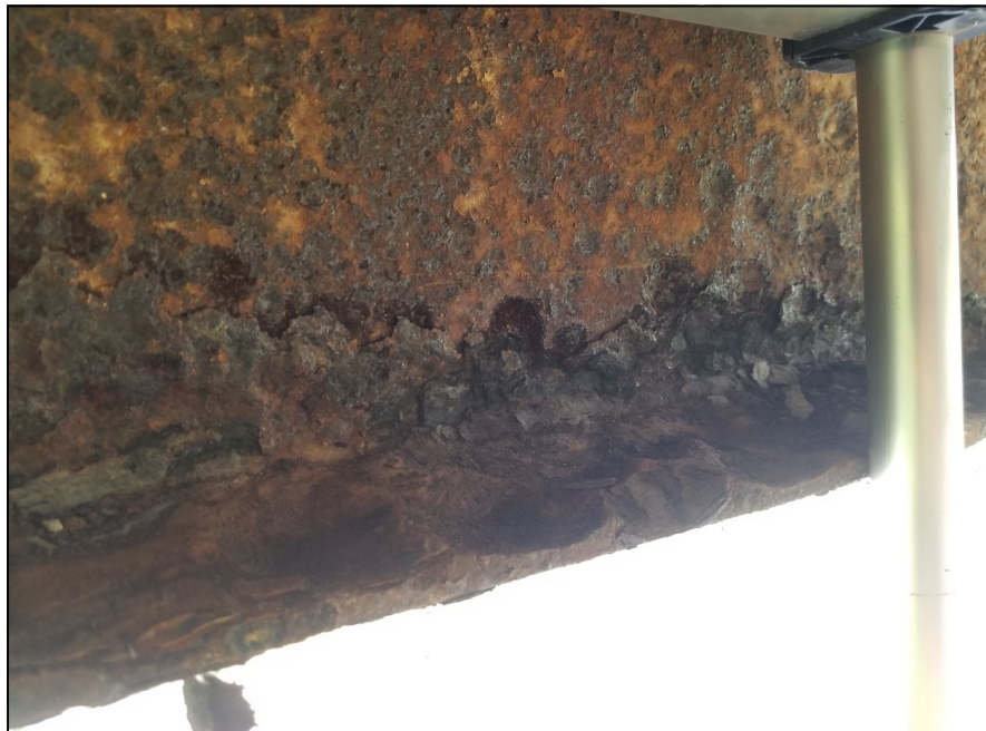
Photo 13 - Approximately 50% section loss at bottom flange of cross beam (September 22, 2020).
