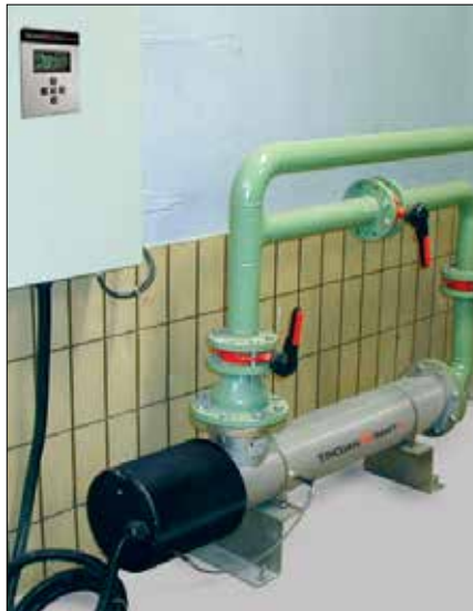
The highly efficient "L-shaped" design and low-pressure, high-output (LPHO) amalgam lamps result in an extremely compact footprint.
