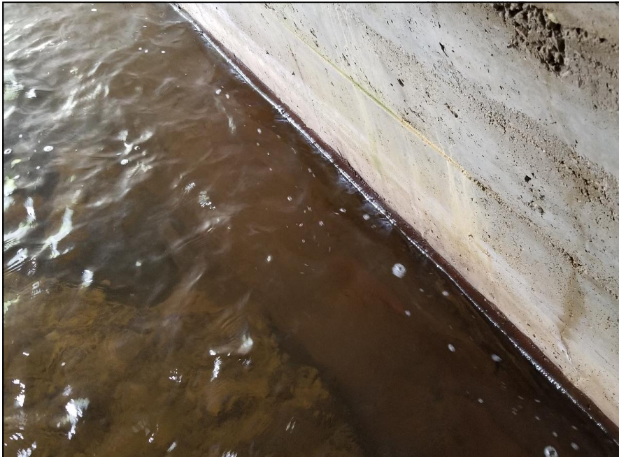
Photo 14 - Top of foundation exposed at southwest.
