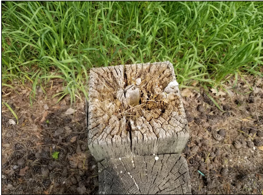
Photo 7 - View of typical rotted post.
