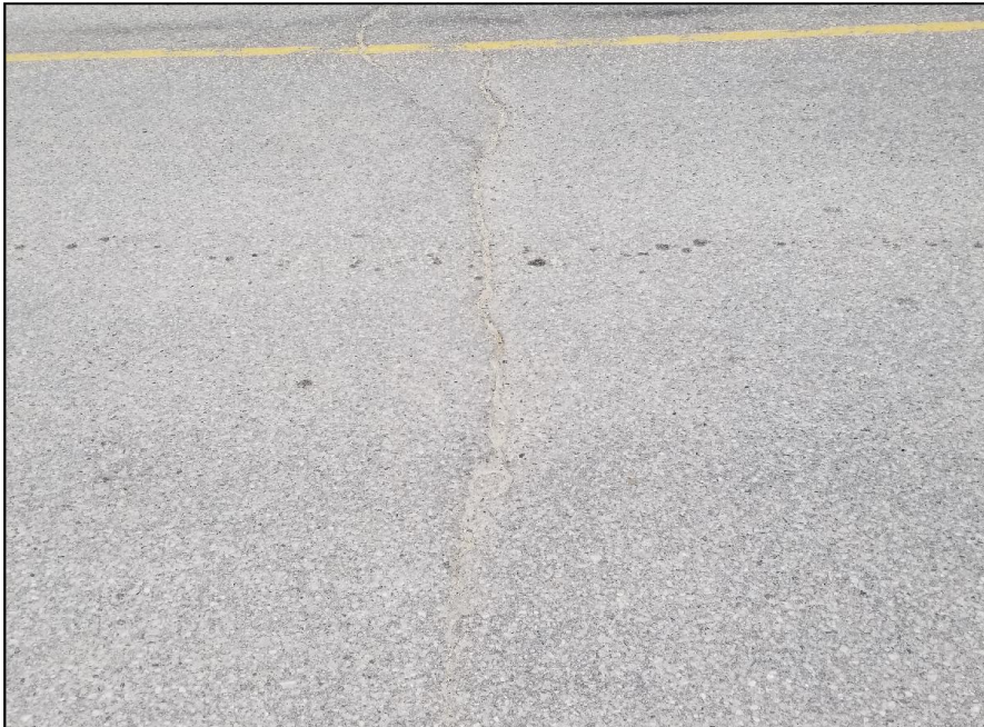
Photo 4 - Typical transverse crack in asphalt.
