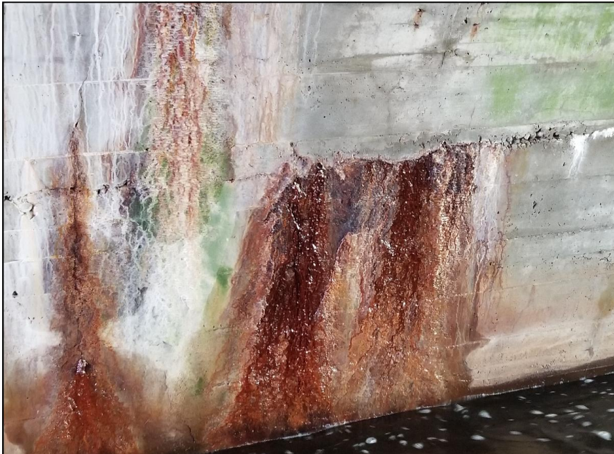
Photo 12 - Active water seepage through barrel wall.
