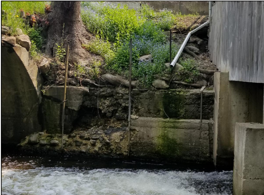
Photo 8 - Deteriorated retaining wall at southeast.
