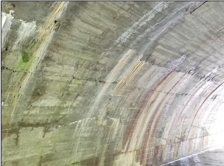
Photo 10 - Evidence of water seepage through original construction joints.
