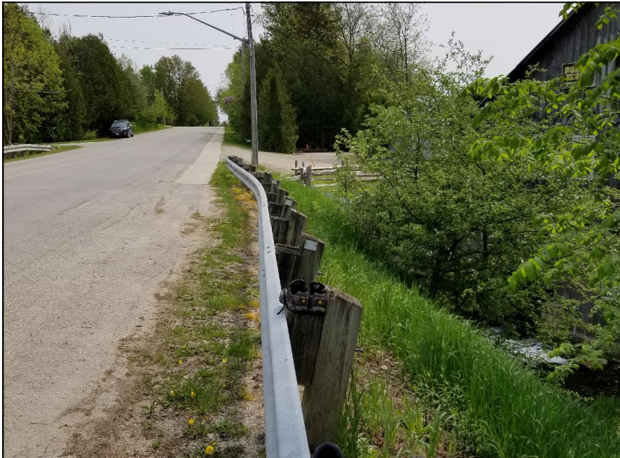
Photo 6 - Outward rotation of south steel beam guiderail.
