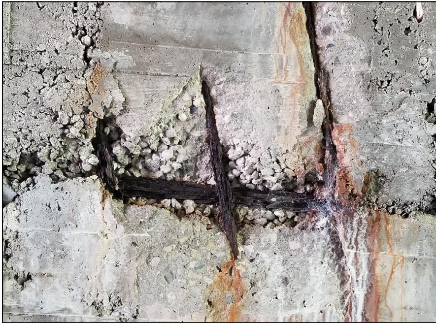
Photo 13 - Exposed reinforcing with severe section loss.
