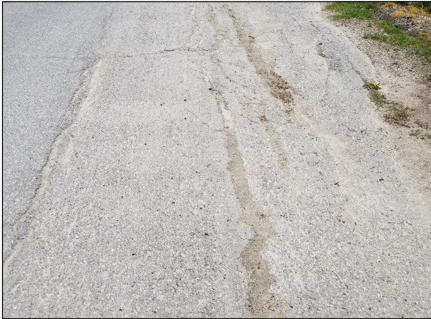
Photo 5 - Settlement and cracking of asphalt along southern edge of wearing surface.
