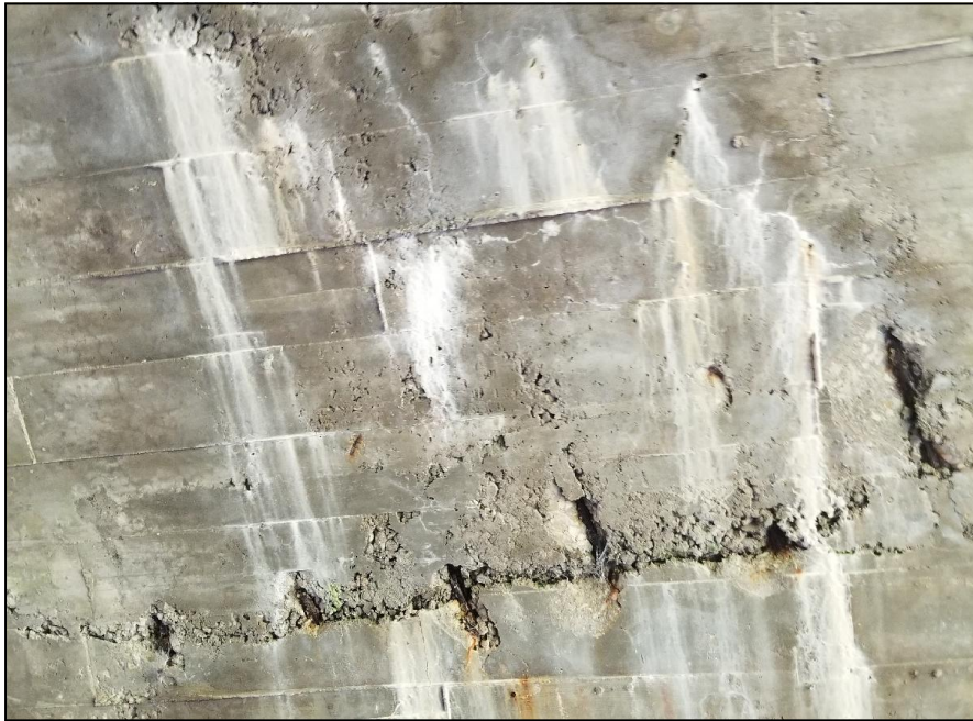
Photo 11 - Barrel wall with exposed reinforcing.
