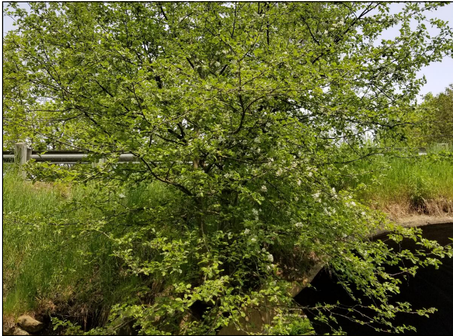
Photo 15 - Large vegetation (tree) growing on top of culvert.
