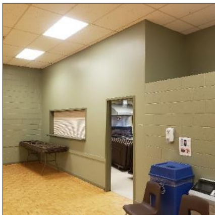
Asbestos-containing drywall joint compound wall, location 2.
