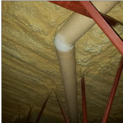
Asbestos-containing paring cement present on a rain water leader pipe fitting, location 2.
