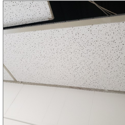
Non-asbestos 24"x48", lay-in, small and medium pinhole ceiling tiles, location 25.
