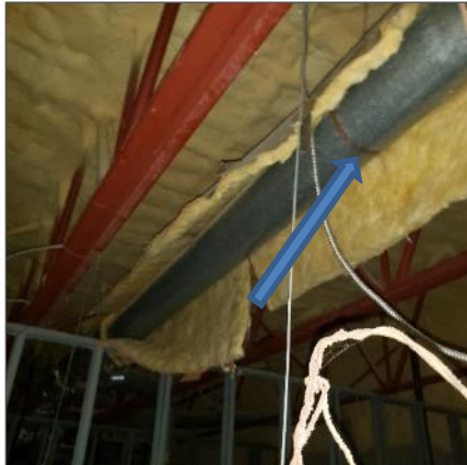
Presumed asbestos-containing brown duct mastic present on fiberglass insulated duct, location 3.
