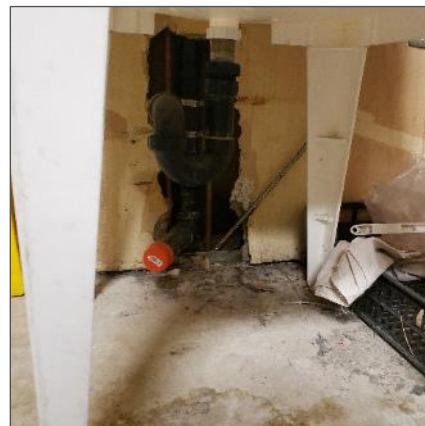
Asbestos-containing drywall joint compound on wall in poor condition with debris, location 9.
