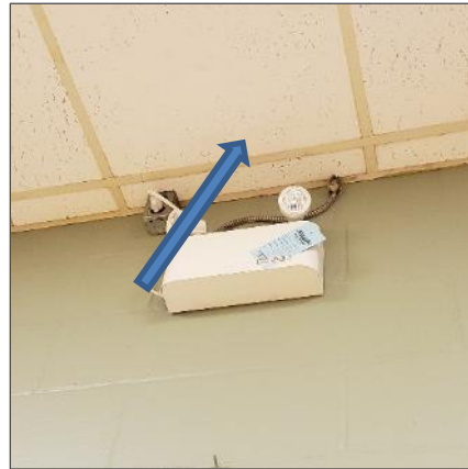
Asbestos-containing 24"x48", lay-in, pinhole and lengthwise fissure, location 2.
