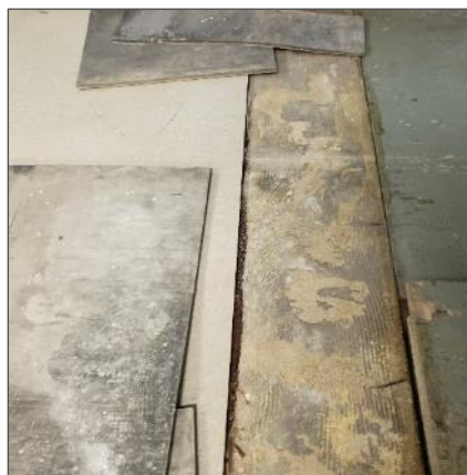
Non-asbestos beige mastic present under grey rubber floor tiles, location 1.
