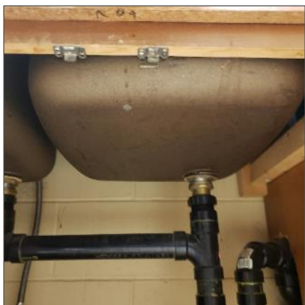
Asbestos-containing gold antisweat mastic present underneath a sink, location 8.
