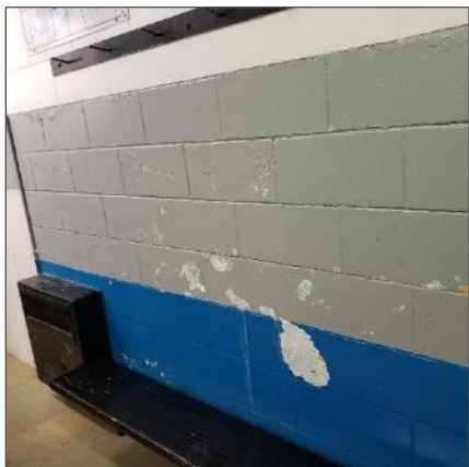
Dark blue paint with elevated levels of lead flaking from concrete block wall, location 13.
