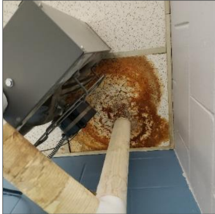
Mould growth and staining present on ceiling tile, location 1.
