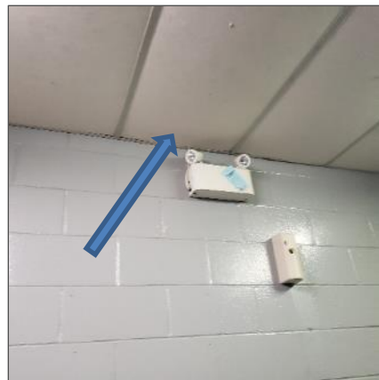
Non-asbestos 24"x48" white wood fibre ceiling tiles, location 24.
