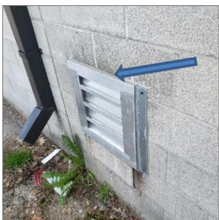
Non-asbestos light grey caulking at exterior vent penetration, location 32.
