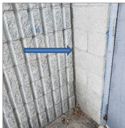
Asbestos-containing grey expansion joint caulking present at the exterior, location 32.
