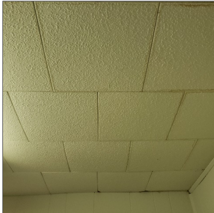
Non-asbestos 12"x12" white textured wood fibre ceiling tiles, location 25.
