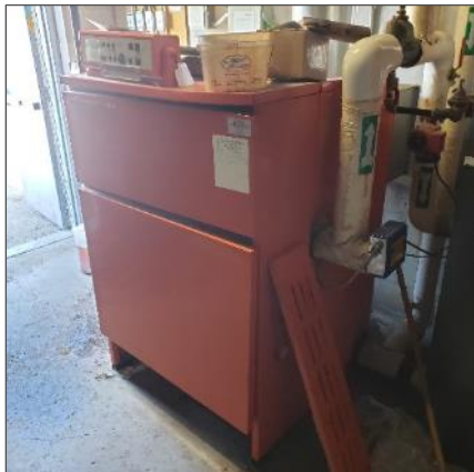
Boiler insulated with non-asbestos fiberglass, location 27.
