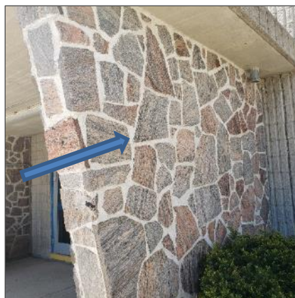
Non-asbestos mortar present in exterior decorative stone wall, location 32.
