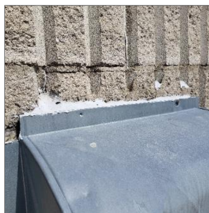
Non-asbestos grey and yellow caulking underneath present at exterior vent penetration, location 32.
