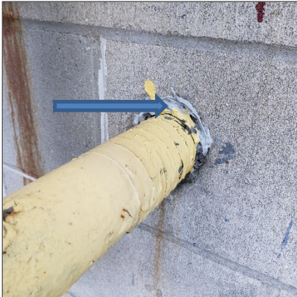
Asbestos-containing grey firestopping present at gas line penetration at the exterior, location 32.
