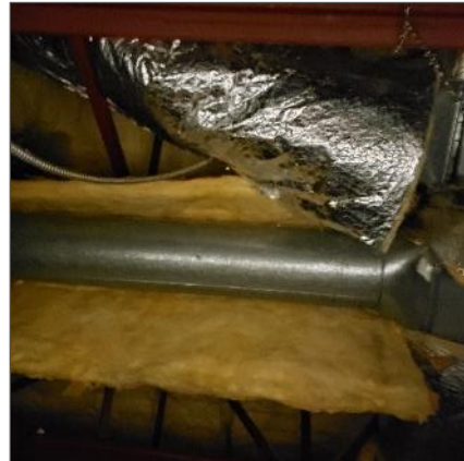
Ducting insulated with foil-faced fiberglass, location 2.
