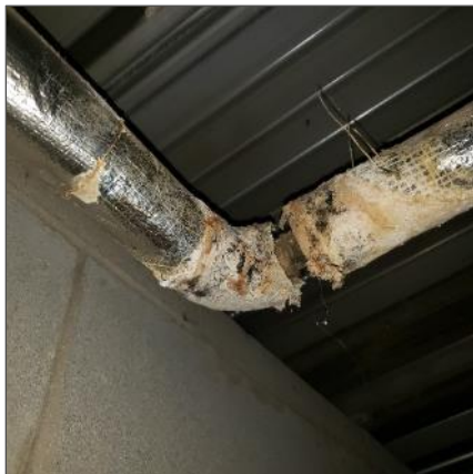
Asbestos-containing paring cement present on a hot water pipe fitting in poor condition, location 1.
