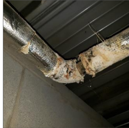
Mould growth present on a pipe fitting with asbestos-containing parging cement, location 1.
