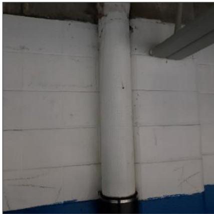
Asbestos-containing Transite rain water leader, location 26.
