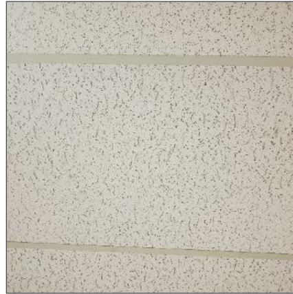
Non-asbestos, 24"x48", lay-in, pinhole and fissure ceiling tiles, location 1.
