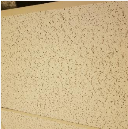
Non-asbestos 24"x48", lay-in, pinhole and width-wise fissure ceiling tiles, location 2.
