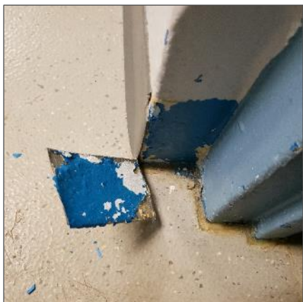
Non-asbestos beige mastic present under grey baseboards, location 1.
