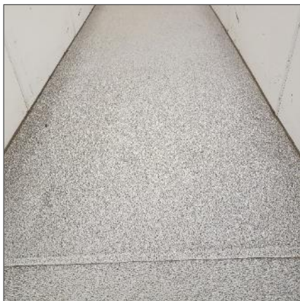
Non-asbestos white and grey pebbled vinyl sheet flooring, Location 31.
