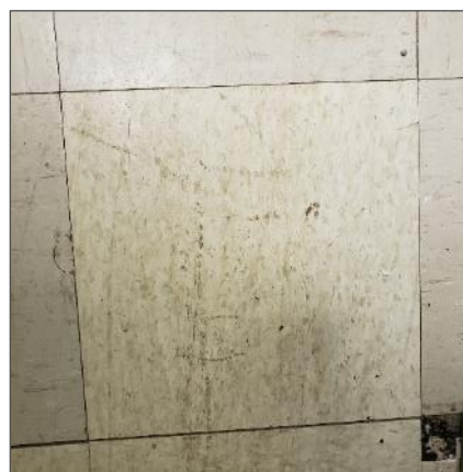
Non-asbestos 12"x12" white, beige and olive fleck vinyl floor tiles with asbestos-containing mastic, location 3.
