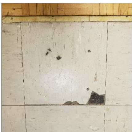
Asbestos-containing 12"x12" light grey with red and white fleck vinyl floor tiles and associated mastic, location 3.
