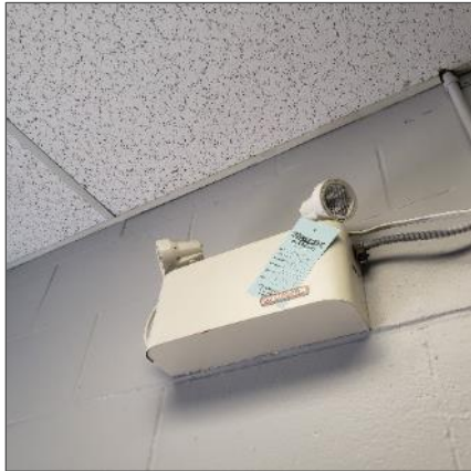
Lead-containing batteries presumed present in emergency lighting, location 1.
