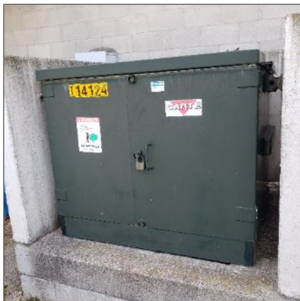
Transformer with presumed PCB containing dielectric fluid present at the exterior, location 32.
