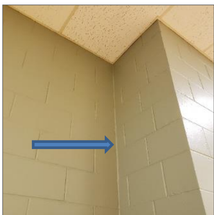
Asbestos-containing white caulking present at interior concrete block expansion joints, location 2.
