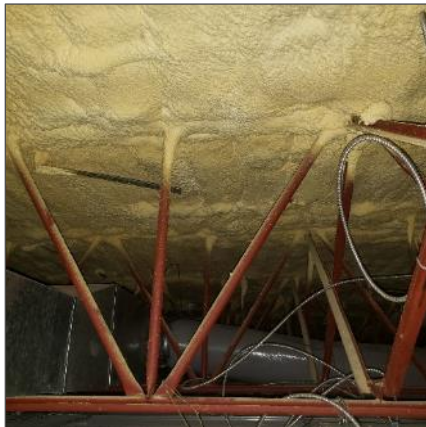
Non-asbestos yellow foam spray-applied insulation present on the structure, Location 2.
