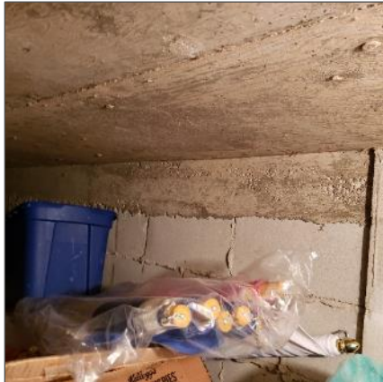
Non-asbestos parge present on concrete walls and ceilings, location 20.
