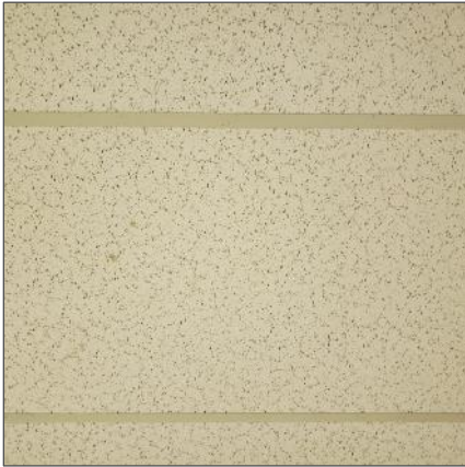
Non-asbestos 24"x48", lay-in, pinhole and fleck ceiling tiles, location 1.
