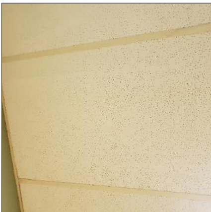
Asbestos-containing 24"x48", lay-in, small and medium perforation ceiling tiles, location 3.
