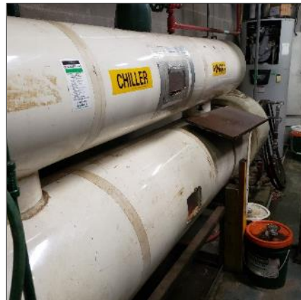
Chiller insulated with non-asbestos fiberglass, location 27.
