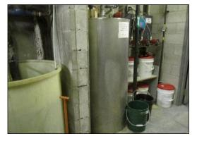
View of the return tank for the ammonia within the mechanical room.
