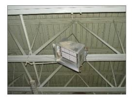
View of a typical gas-fired unit heater in the grandstand of the arena.
