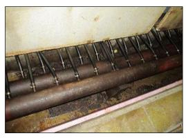
View of the refrigerant manifold for the cooling of the rink slab.
