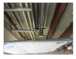
View of the infrared gas-fired tube heater located in the ice resurfacing room.
