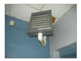
View of a typical hydronic unit heater within the Site Building.
