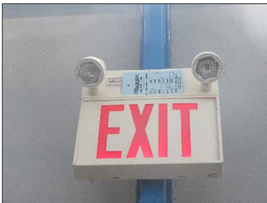
Illuminated exit signage and emergency lighting noted throughout the Site Building.
