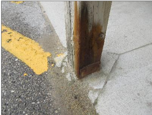
View of stained wood columns serving the east metal canopy.
