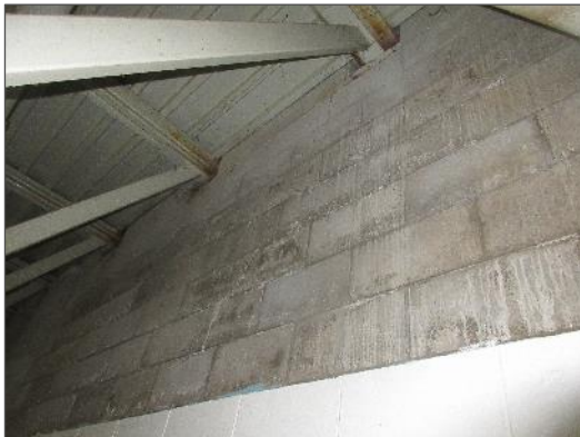
View of efflorescence noted at the upper portions of the walls within the rink areas.
