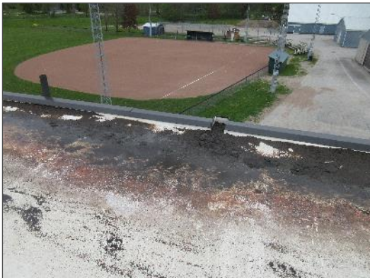
View of typical organic growth noted throughout the roof.
