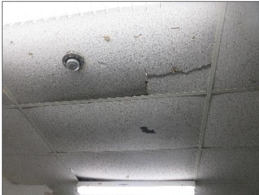
View of typical bowing and damaged ceiling tiles noted within the various change rooms of the Site Building.
