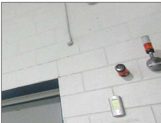
Emergency audio and visual fire alarm observed.
