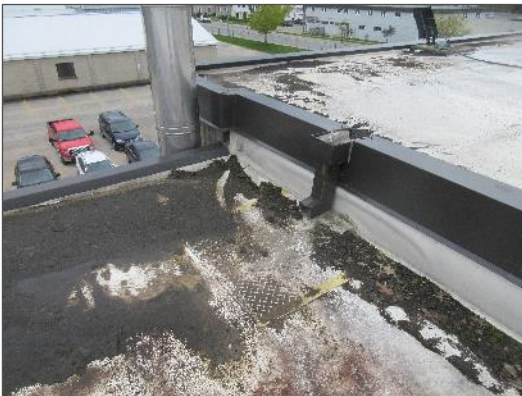
View of a scupper and downspout draining to the lower level.
