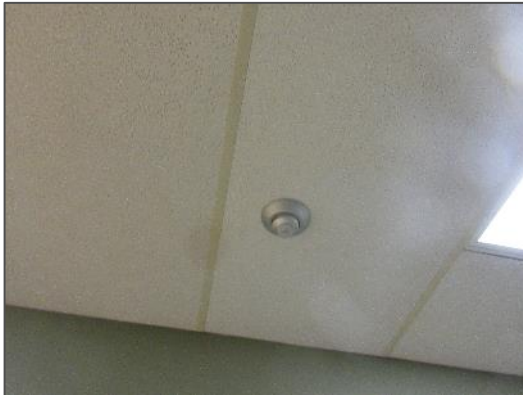
View of a typical heat and smoke detector noted within the Site Building.
