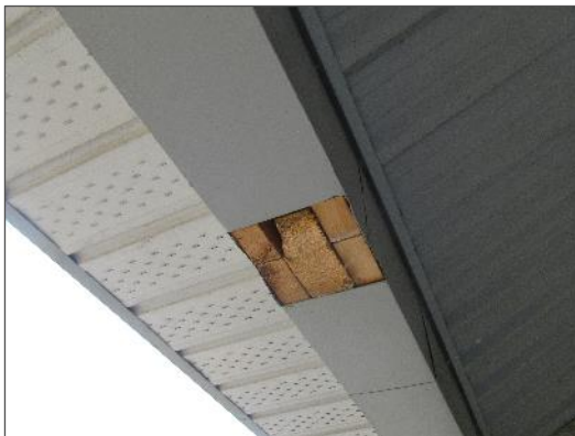
View of missing soffit at the east metal canopy.
