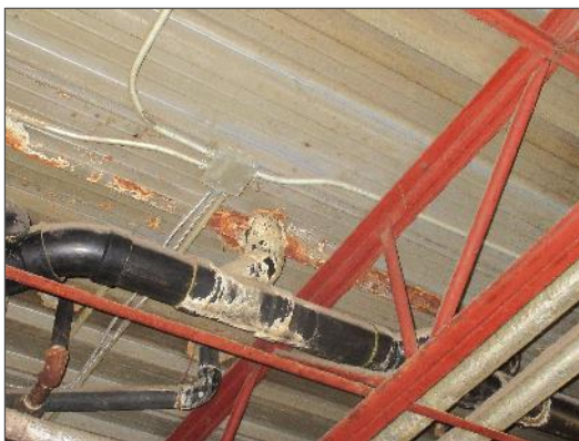
View of an area of isolated corrosion noted within the change room.
