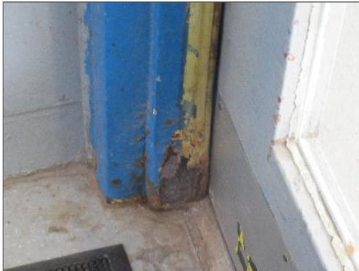
View of typical corrosion noted at the base of the main entrance door frame.
