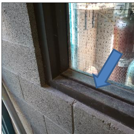
Asbestos-containing grey/black butyl tape present around the boiler room window frame, location 1.
