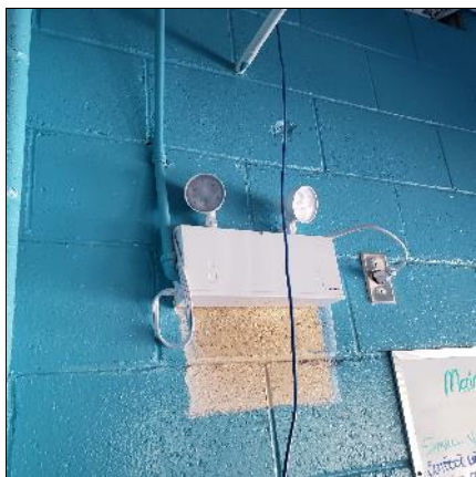
Lead-containing batteries are presumed present in the emergency lighting in the family change room, location 4.
