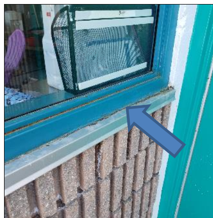
Non-asbestos black caulking present around the exterior window frames of the guard house, location 10.
