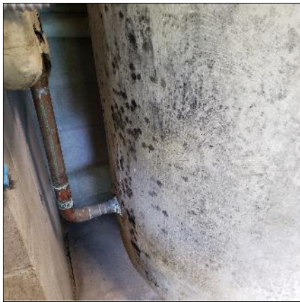
Visible mould growth present on the boiler canvas in the boiler room, location 1.
