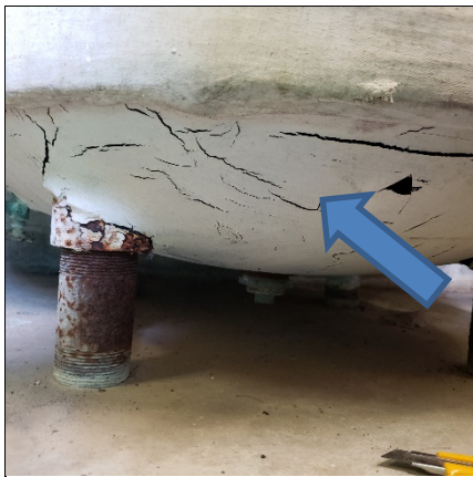
Non-asbestos black insulation present on underside of the boiler, location 1.
