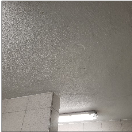
Non-asbestos stippled texture finish present on the ceiling in the men's washroom shower, location 3.
