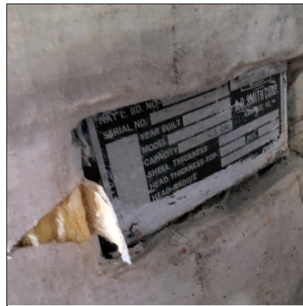
Non-asbestos fibreglass insulation present on face of boiler, location 1.
