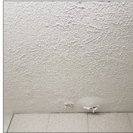
Non-asbestos swirling texture finish present on the ceiling in the women's washroom shower, location 7.
