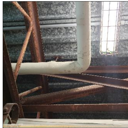
Visible mould growth present on the pipe canvas in the boiler room, location 1.
