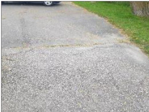
View of cracking noted within the asphalt paved parking areas on the lower, central portion of the Site.
