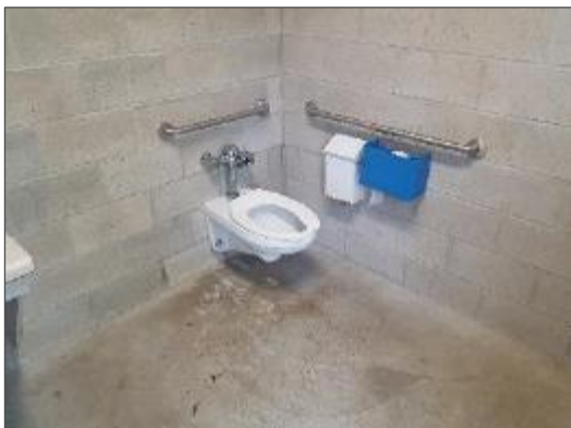
View of staining at the cast-in-place concrete slab noted within the washroom spaces of the splash pad outbuilding.
