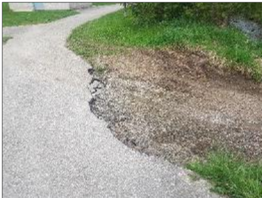
View of deteriorated asphalt pavement walkway within the central portion of the Site.
