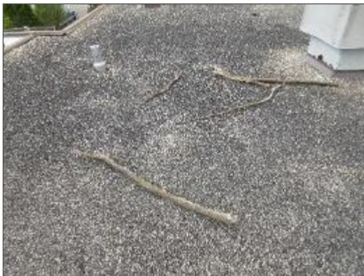
View of debris noted atop the BUR system at the Site Building.
