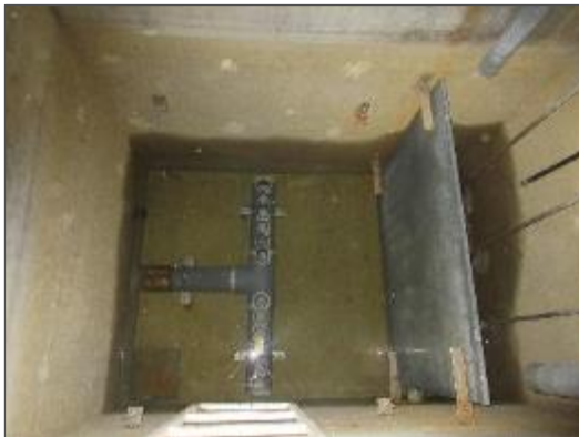
View of the in-ground water treatment tank noted serving the pool.
