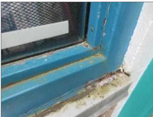
View of missing sealant noted at the SG window systems.
