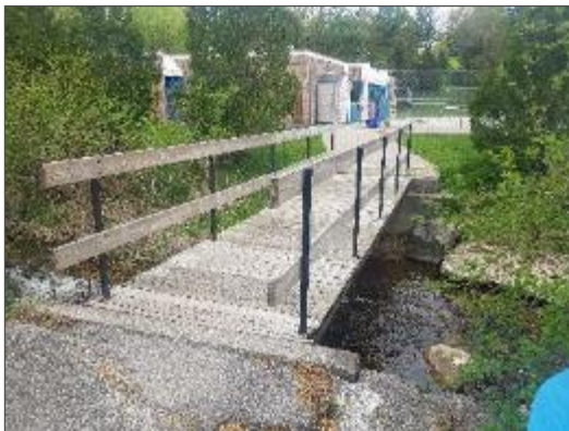
View of the steel and wood framed bridge noted crossing the stream which flows across the centre of the Site. (Not included in assessment)
