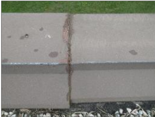
View of deteriorated sealants noted at perimeter metal flashing.
