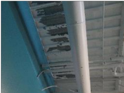
View of peeling paint noted at the underside of the steel decking of the Site Building.
