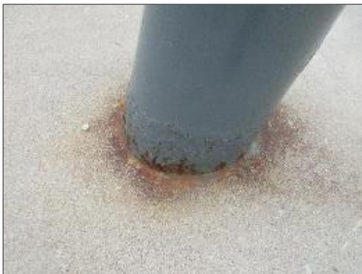
View of minor corrosion noted at the base of the diving boards.
