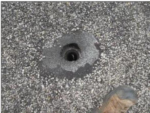
Typical roof drain missing roof drain strainer.
