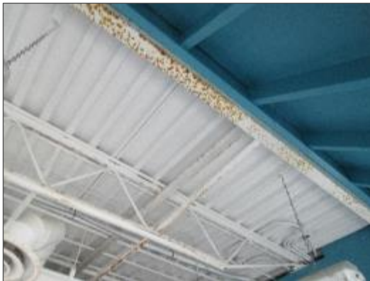
View of corrosion noted at the underside of the steel decking of the Site Building.
