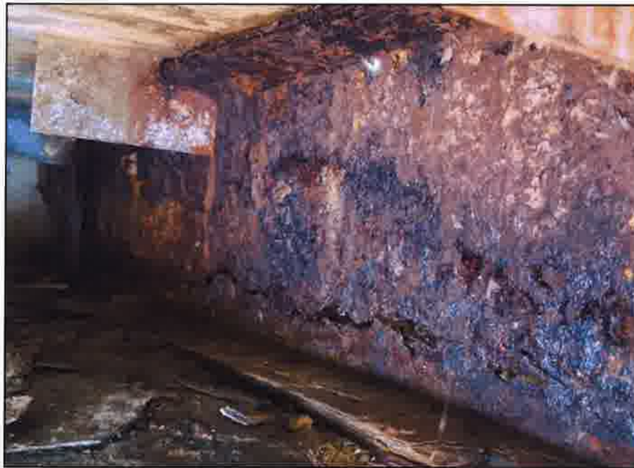
Photo 7 - View of severely corroded stringer end at west.
