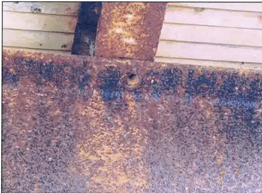
Photo 8 - View of sheared bolt floor beam to stringer connection.
