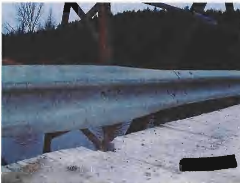
Plate 4 Vertical web members are damaged at just above the deck (south east web member shown). The steel guard is not attached to the structure at this location.
