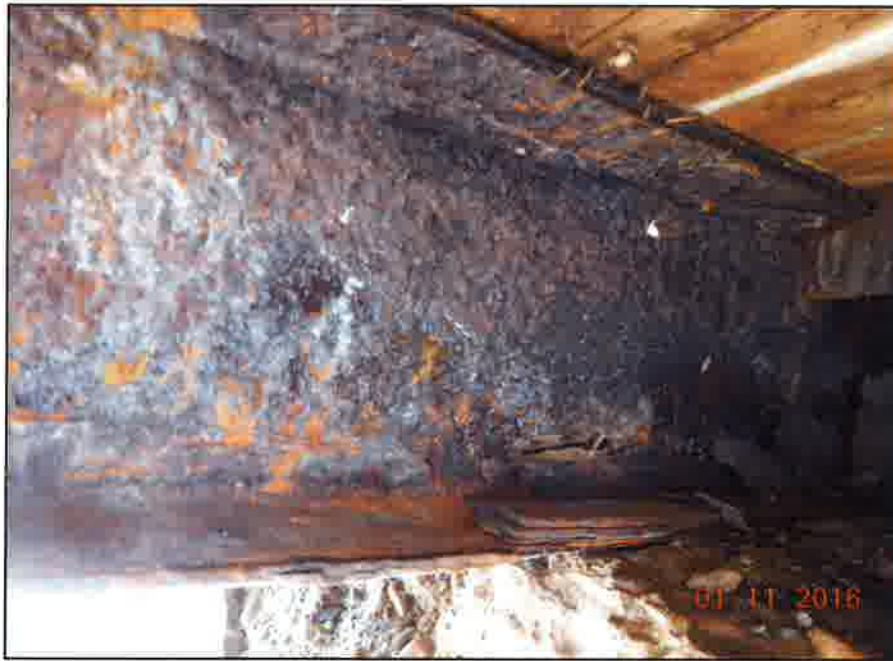
Photo 5 - View of deteriorated steel stringer.
