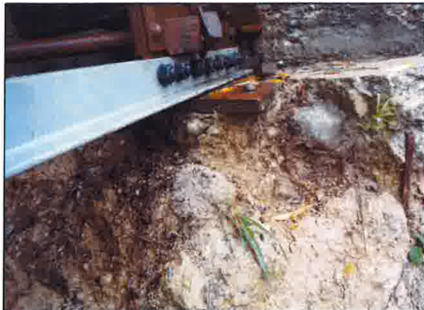
Photo P-6- View of spalled abutment at truss bearing.
