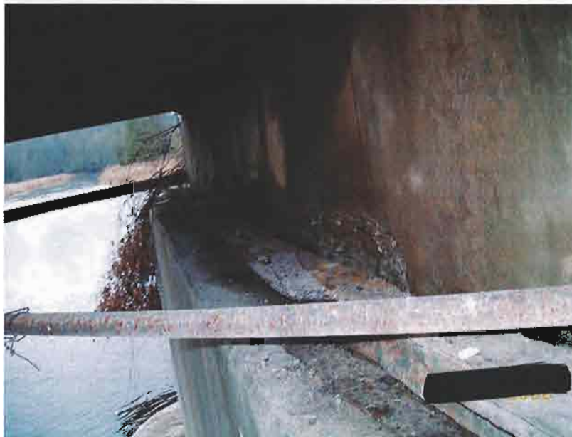
Plate 8 The bottom chord cross tie over the west abutment has corroded and is losing area.
