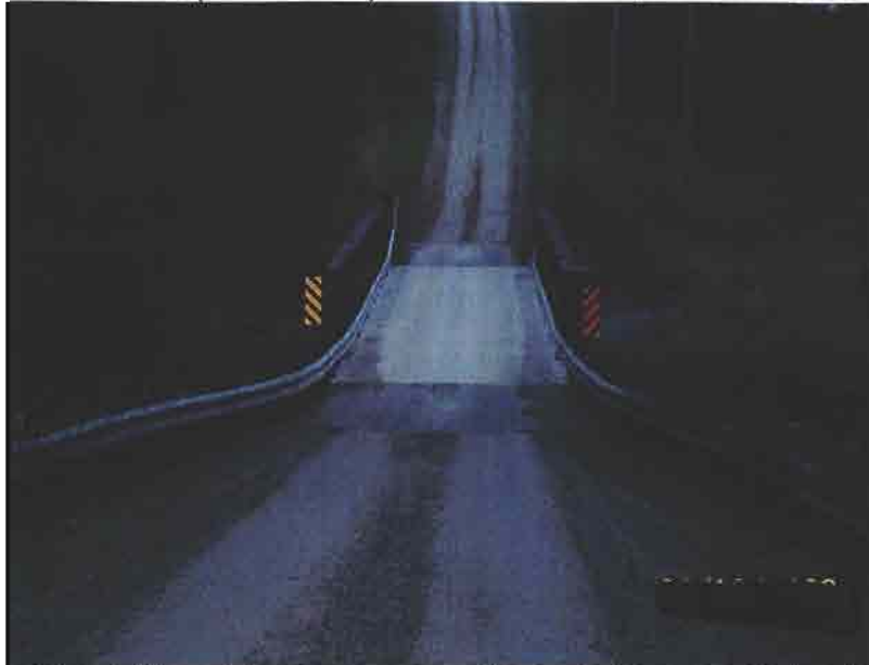
Plate 1 View of the structure from the west. Note that the south truss appears to be out of alignment.
