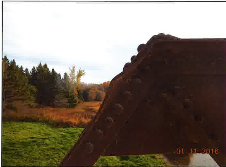
Photo 7 - View damaged steel plate at southeast corner of truss.
