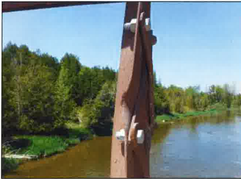
Photo 7 - View of recently replaced web member with impact damage
