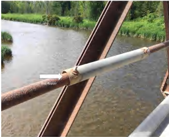
Image 14: Railing Repairs North Side of Bridge
