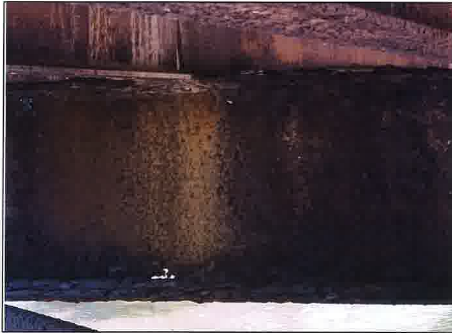
Photo 9 - View of severe corrosion with perforations at east floor beam.
