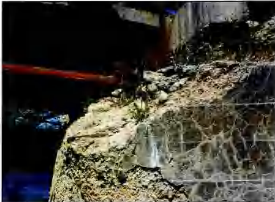
Photo 6 - View of spalled abutment at truss bearing.
