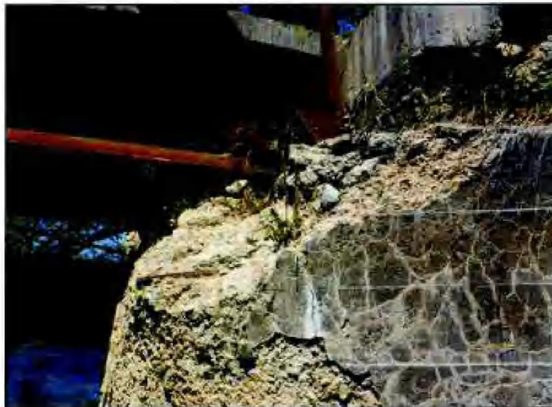
Photo 6 - View of spalled abutment at truss bearing.
