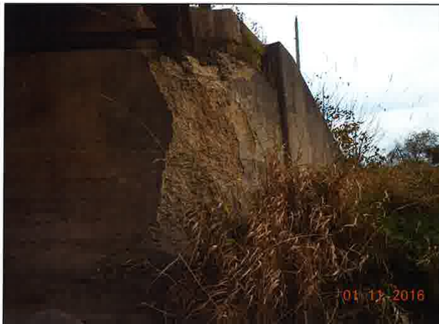
Photo 10 - View of spalled concrete on east wing wall
