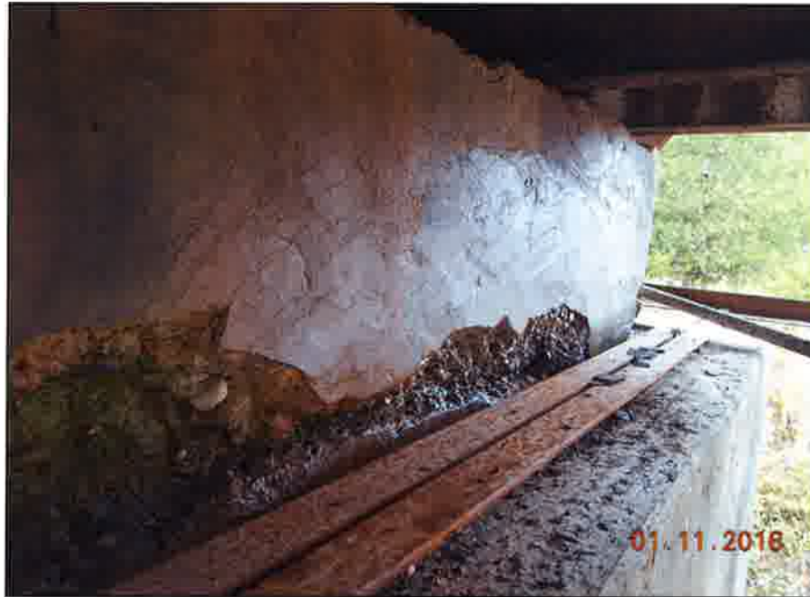
Photo 11 - View of deterioration on west abutment.
