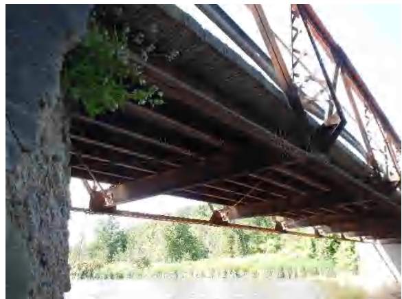
Image 12: Concrete Deterioration on Abutment
