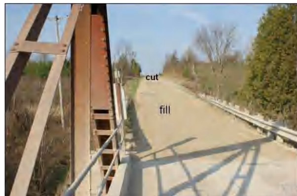
Image 14. Cut western approach to 12 th of Brant Bridge
