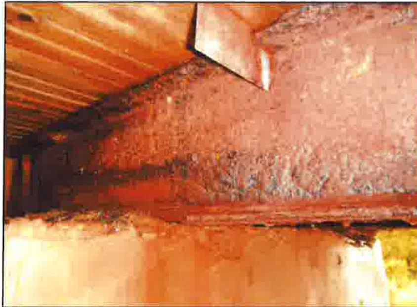
Photo P-7 - View of typical floor beam corrosion at bearing.
