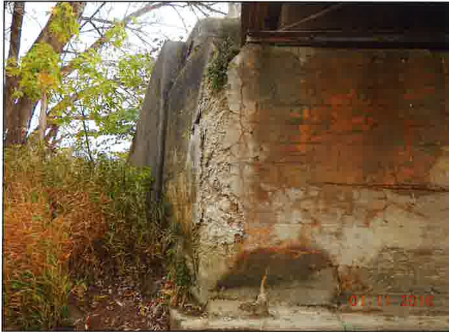
Photo 9 - View of cracking and deterioration on east abutment.
