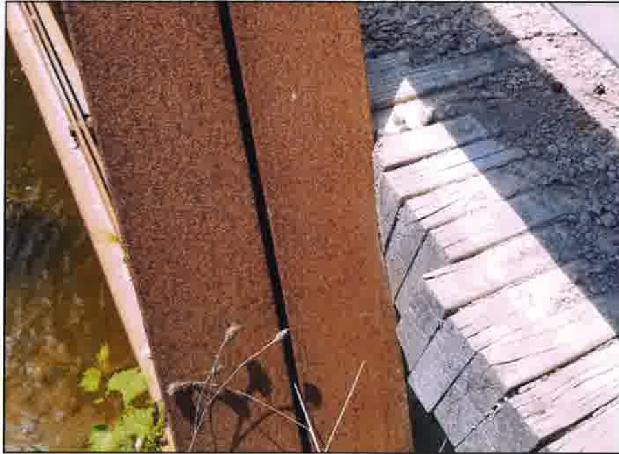
Photo 5 - View of top chord at south pressing against deck top.
