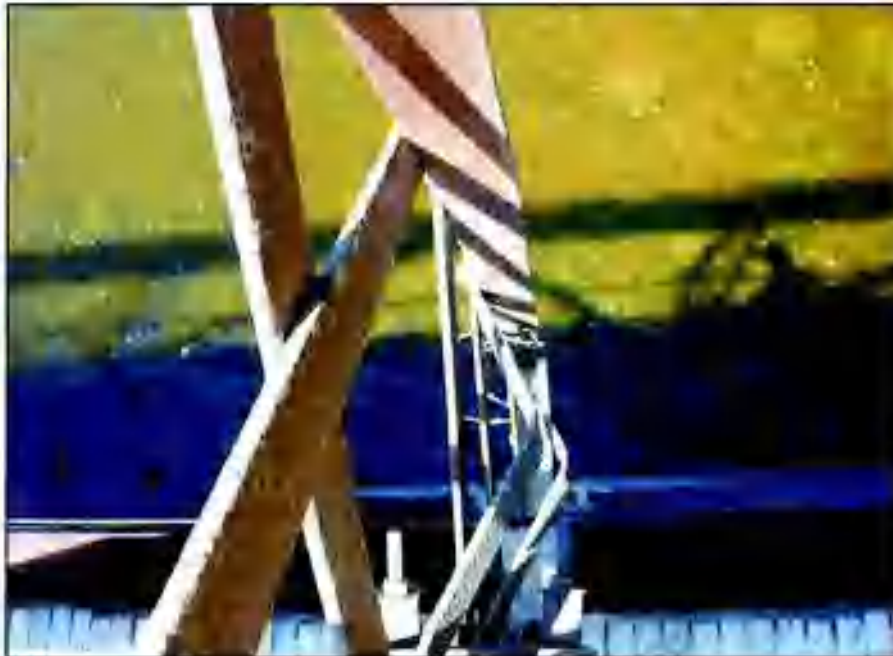
Photo 4 - View of damaged truss lattice.
