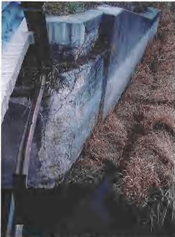
Plate 6 The south east abutment has severely spalled.
