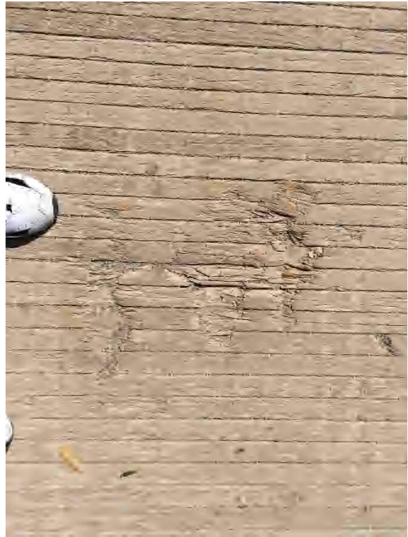
Image 12: Concrete Deterioration on Abutment
