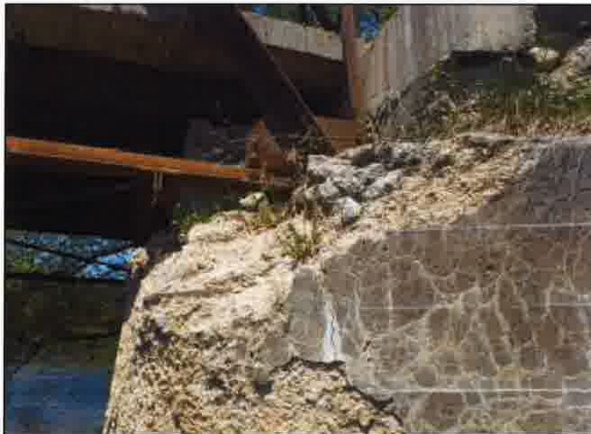
Photo 6 - View of spalled abutment at truss bearing.
