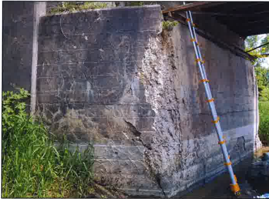
Photo 11 - View of severe spalling with vertical cracks at northeast wingwall.
