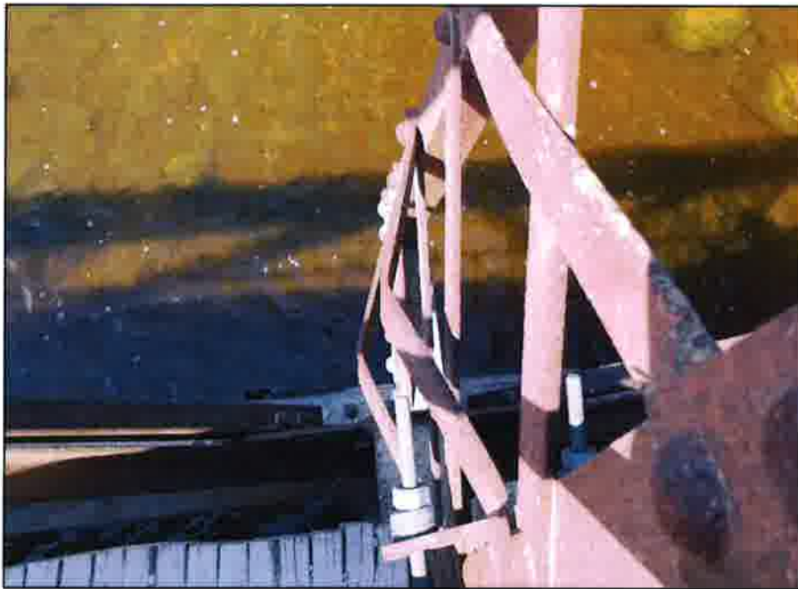
Photo 4 - View of damaged truss lattice at north.
