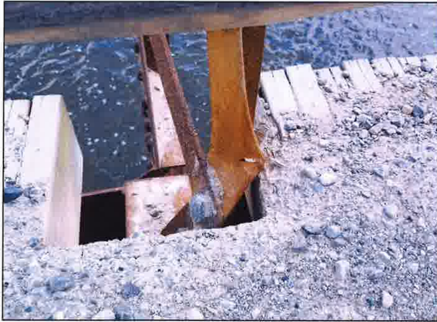
Photo 3 - View of damaged vertical truss support at south.
