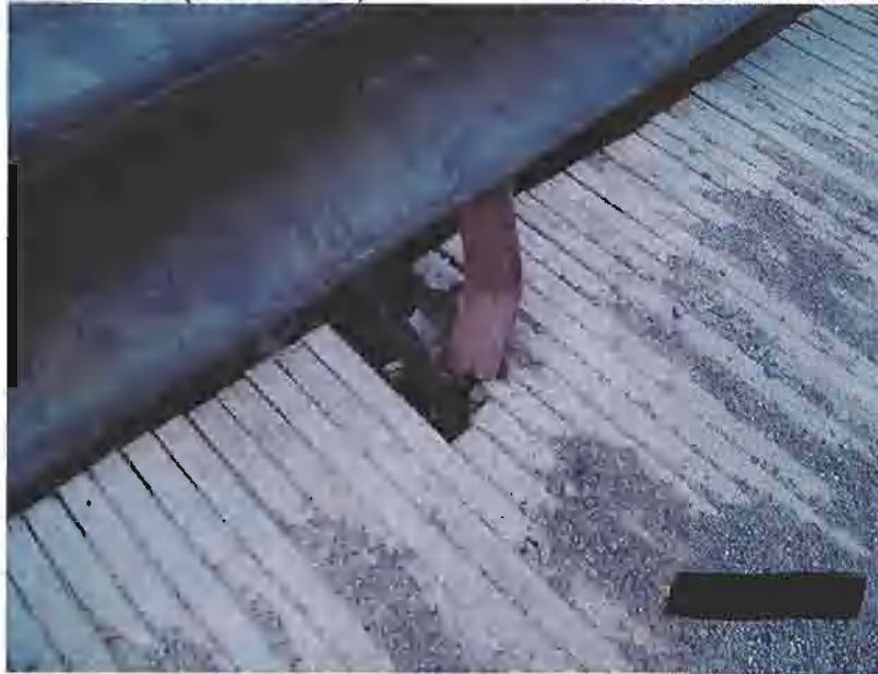
Plate 5 The west vertical web member is completely broken on the south truss.
