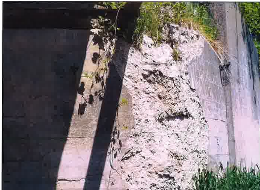
Photo 10 - View of severe scaling and spalling at east abutment.
