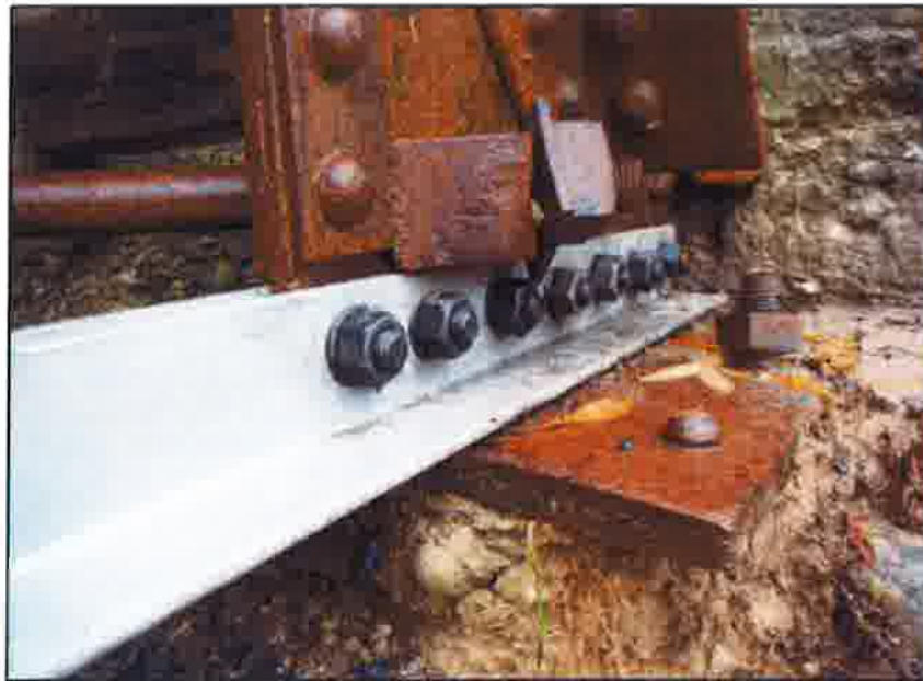
Photo P-5 - View of replaced bottom chord member.
