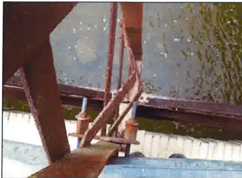
Photo P-4 - View of damaged truss lattice.
