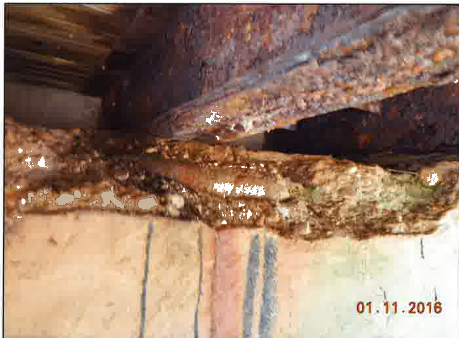
Photo 6 - View of deteriorated steel stringer and west bearing seat.
