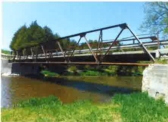
Warren Steel Pony Truss Bridge (Single Span of 30.9 meters).
