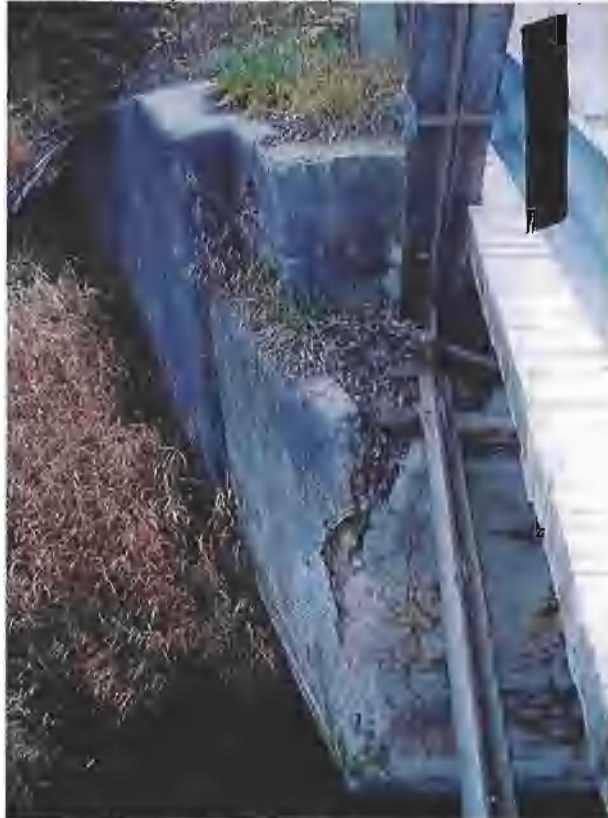
Plate 7 The north west abutment is severely cracked and spalled at the bearing seat. Note also lots of cracking in the north abutment face, which is delaminating.
