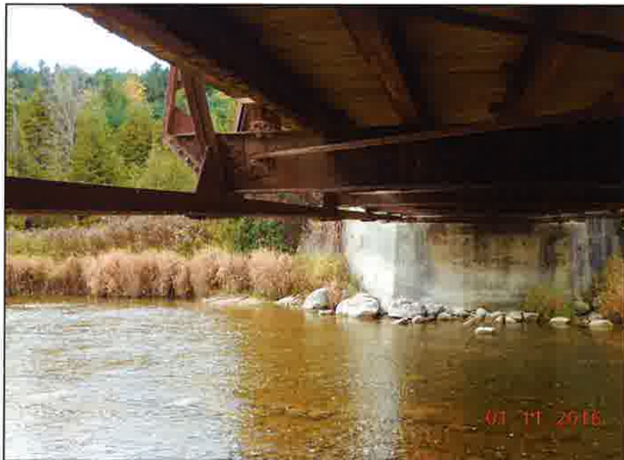
Photo 8 - View of steel floor beams
