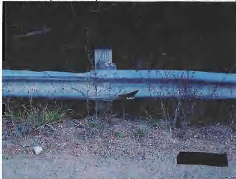
Plate 3 The approach guards are damaged due to impact (north west approach guard shown).
