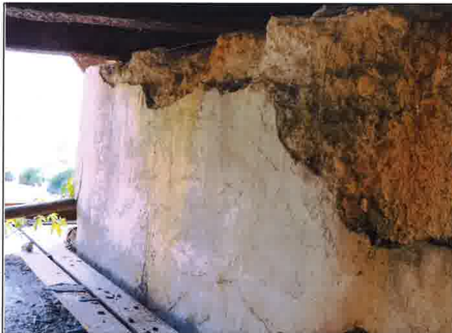
Photo 12 - View of concrete spalling at west bearing seat.
