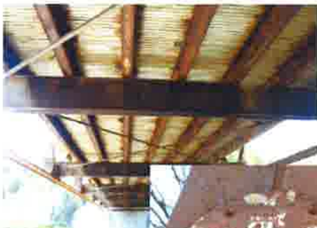
Steel floor beams and stringers supporting a wood deck.
