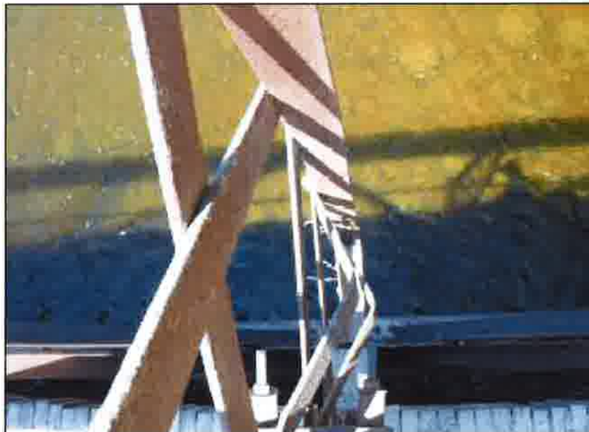
Photo 4 - View of damaged truss lattice.
