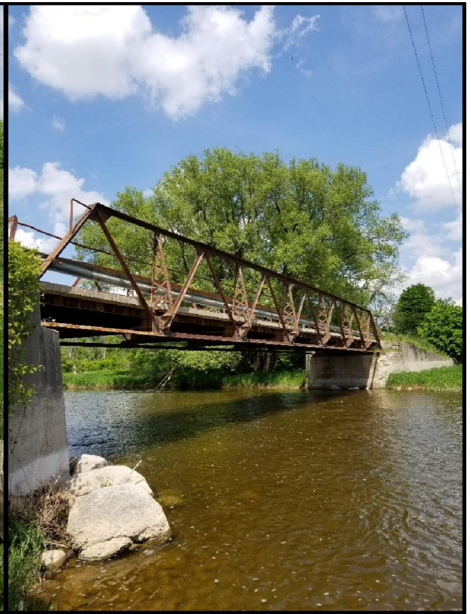
Photo 2: Image showing the single lane steel pony truss bridge.
