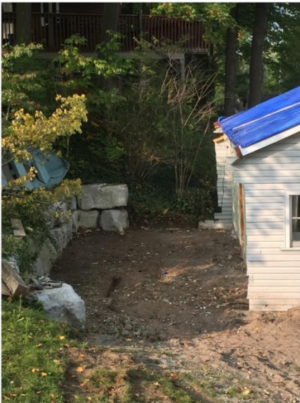
These two pictures show the aftermath of the demolition when they removed the back end of the Bunkie. You can see in the second picture the foundation which was the corner of the old building. Note that the original building was at least 3 – 4 feet from the retaining wall. The width from the New structure to the wall is approximately 1 – 2 feet
