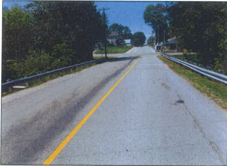
Photo 1 - View of structure from east.
