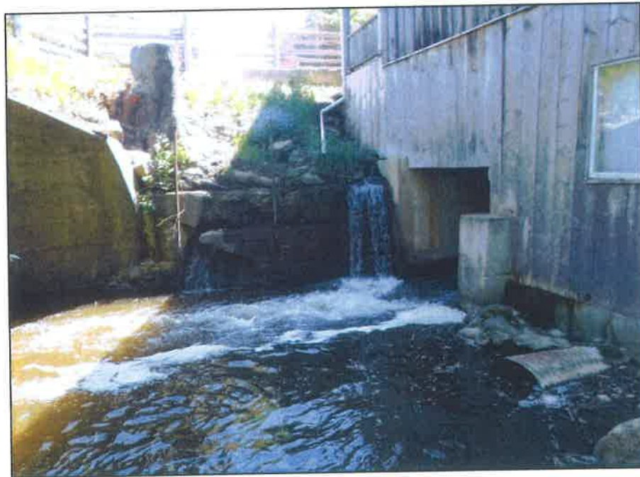
Photo 4 - View of southeast retaining wall.
