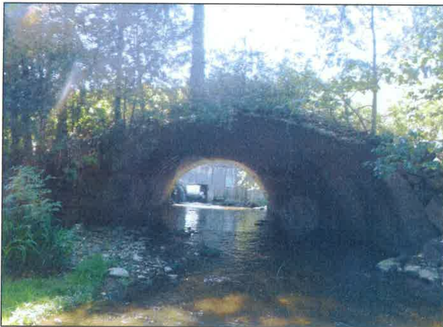
Photo 2 - View of structure from northwest.
