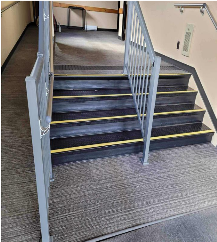
Completed main entrance
