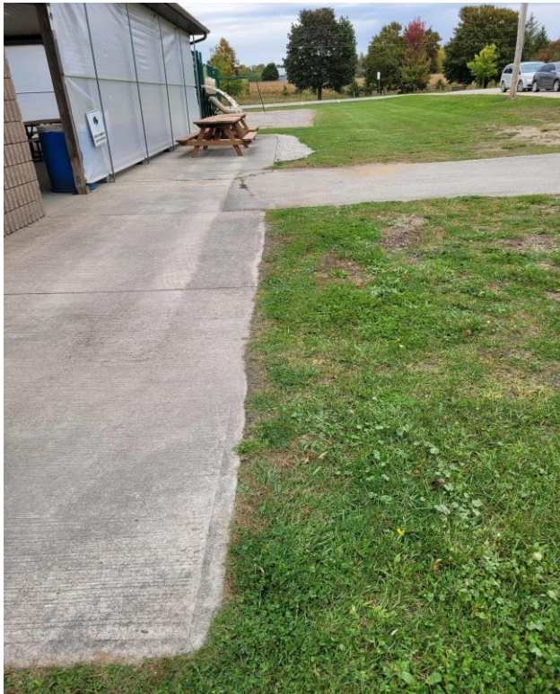
Slope towards the Pavillion
