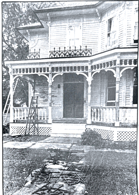
IRON CRESTING , lying on the sidewalk leading to the front veranda, waits to be installed along the top of the veranda. When Sandra Pitt bought the property in January 1986, removal of the thorn hedge surrounding the property was the first thing done.
