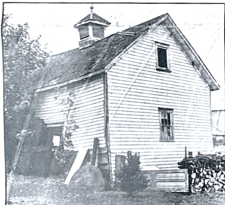
THE CARRIAGE HOUSE , located north west of the house, will be restored in the future. Other future work on the property includes repainting the home to its historical colors and masonry work on the house's foundation.
