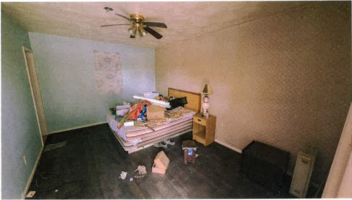
Photo 8: Indoor Observation, two storey building.
