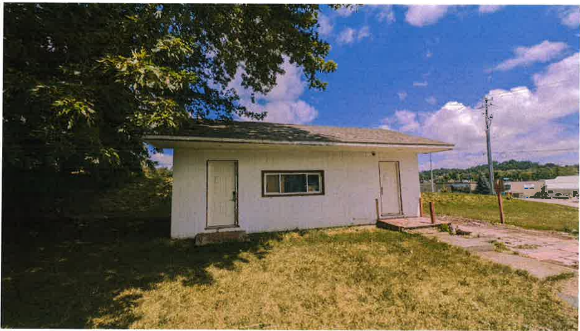
Photo 15: Outdoor observation, south side of the single storey building.
