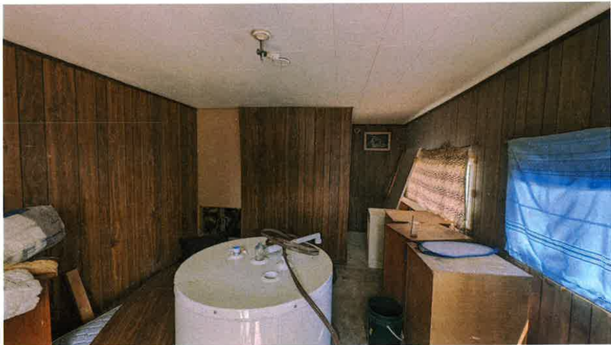
Photo 11: Indoor Observation, single storey building.
