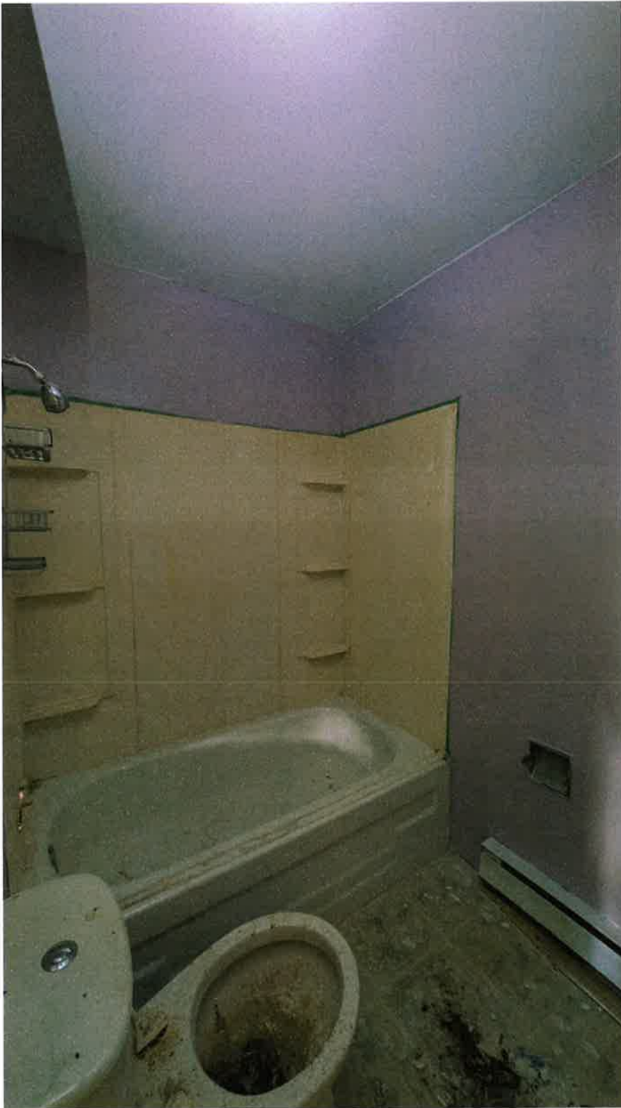
Photo 14: Indoor Observation, single storey building.
