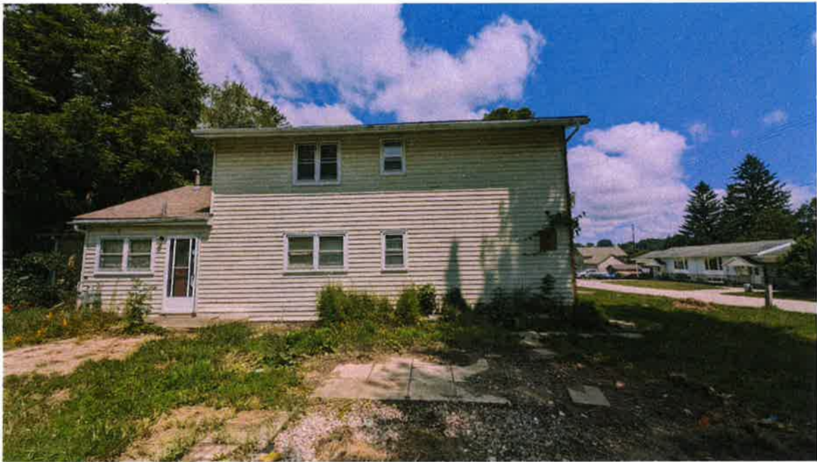
Photo 33: Outdoor observations, south side of the two storey building.
