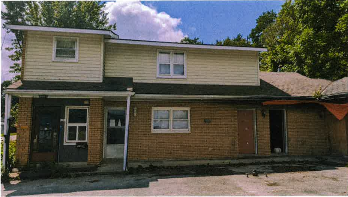
Photo 29: Outdoor observation, north side of the two storey building.
