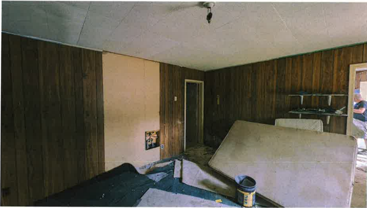
Photo 13: Indoor Observation, single storey building.
