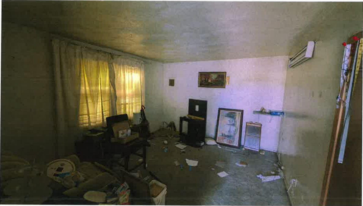
Photo 1: Indoor Observation, two storey building.
