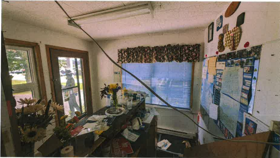
Photo 2: Indoor Observation, two storey building.
