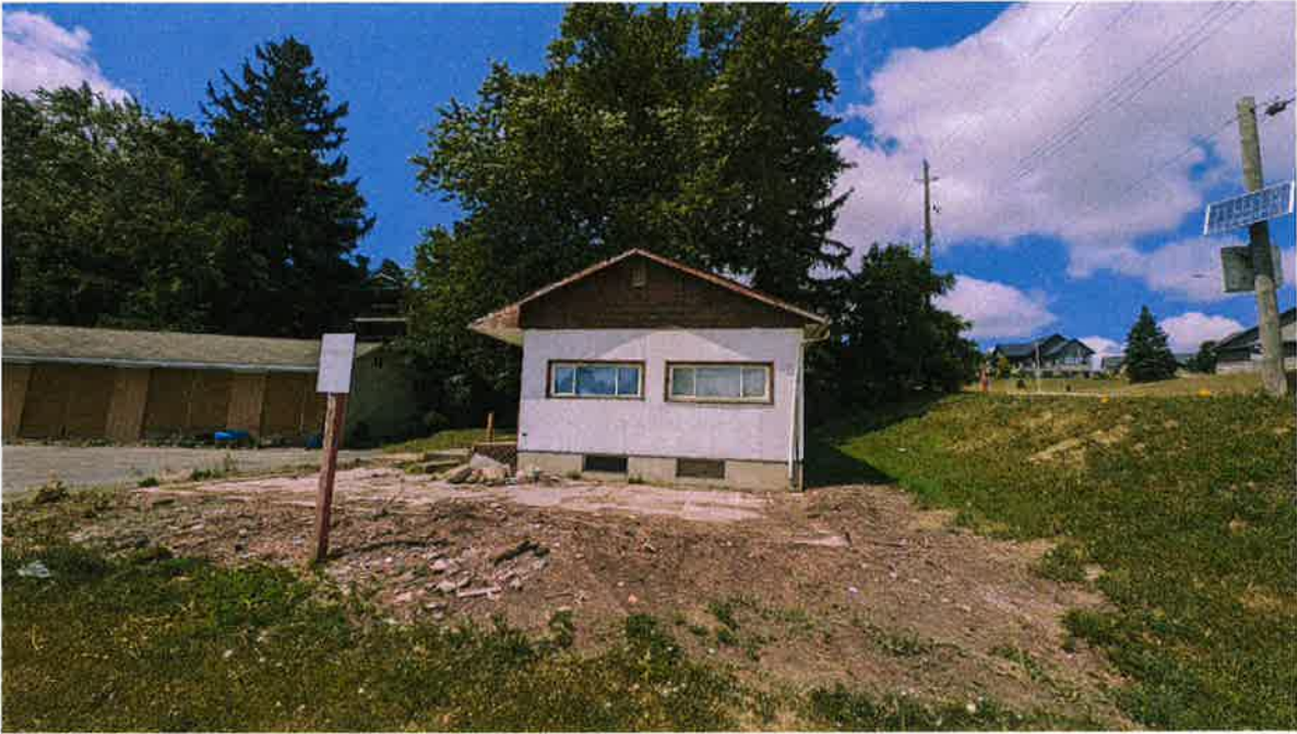
Photo 17: Outdoor observation, east side of the single storey building.
