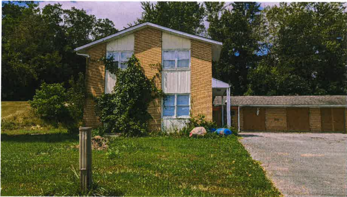
Photo 28: Outdoor observation, east side of the two storey building.
