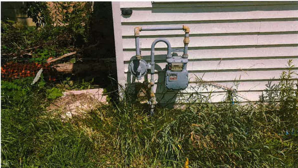
Photo 34: Outdoor observations, south side of the two storey building.
