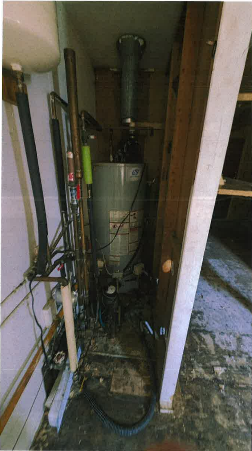
Photo 7: Indoor Observation, two storey building.
