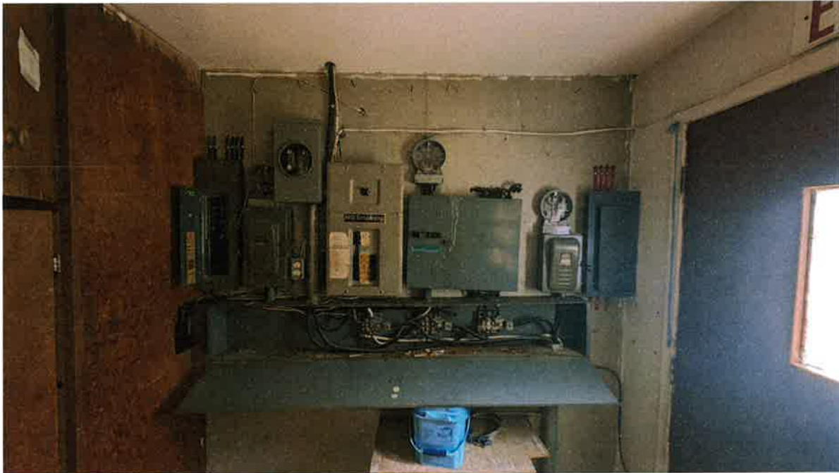
Photo 6: Indoor Observation, two storey building.
