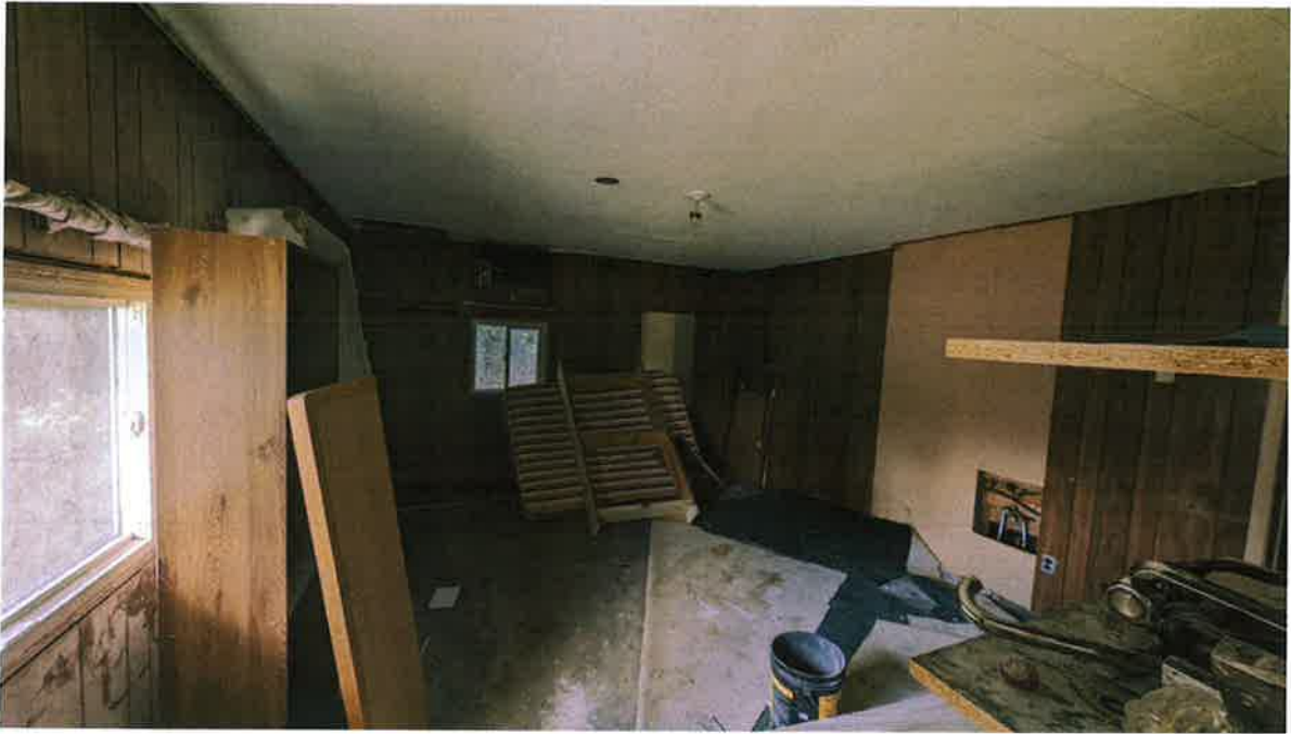
Photo 12: Indoor Observation, single storey building.
