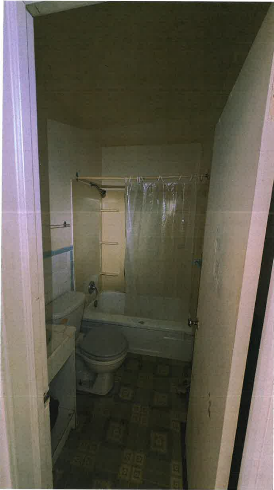
Photo 9: Indoor Observation, two storey building.
