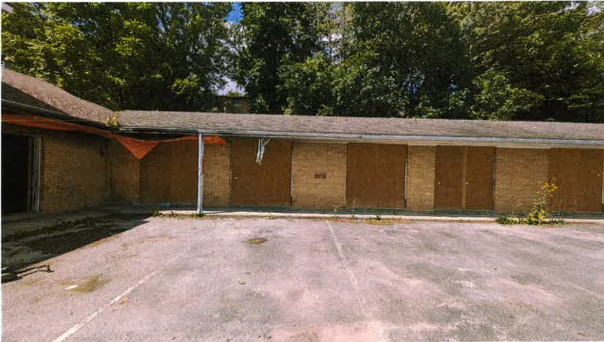
Photo 30: Outdoor observation, east side of the two storey building.
