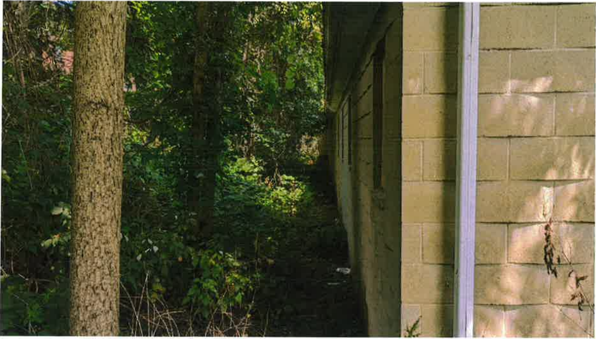
Photo 35: Outdoor observations, west side of the two storey building.
