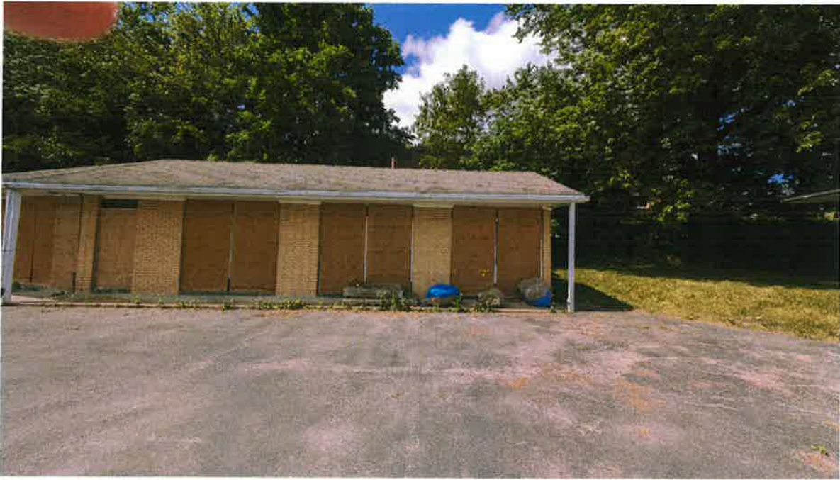
Photo 27: Outdoor observation, east side of the two storey building.
