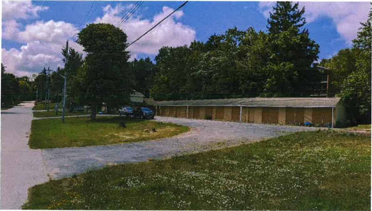
Photo 23: Outdoor observation, east side of the two storey building.
