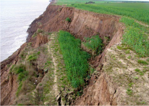
Figure 6 Irregular slope surfaces, slumps, scarps, bumps, bulges
