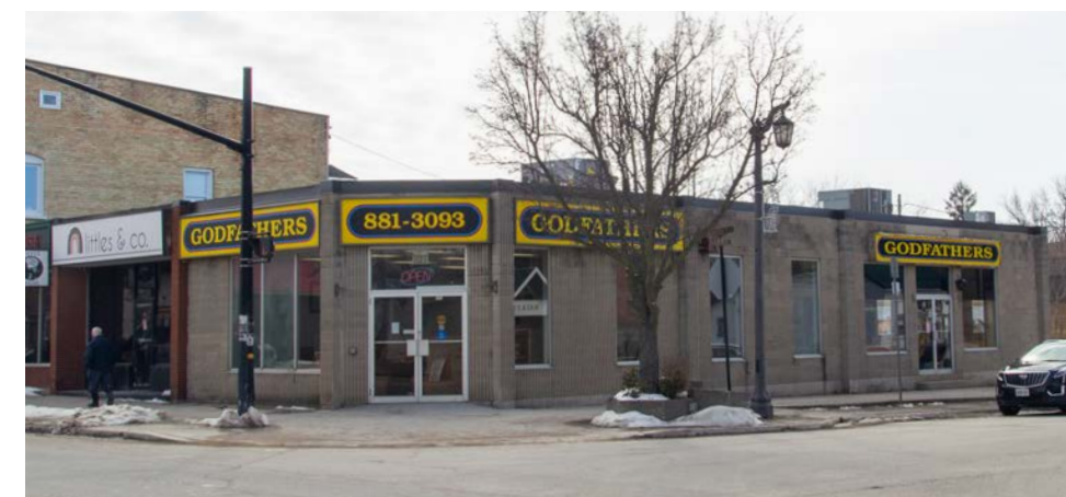
Existing Façade, March 2023
