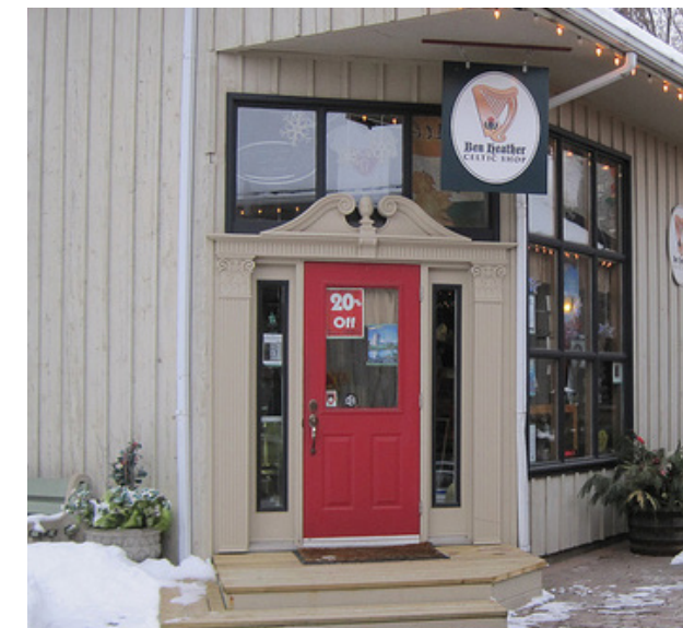
Board and batten exterior
