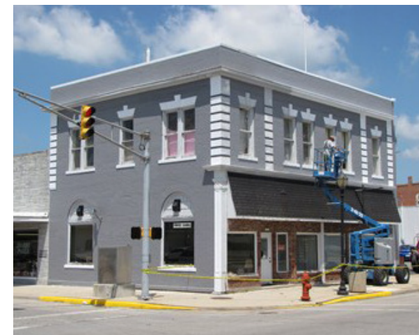
Painted brick preserves and highlights historical character
