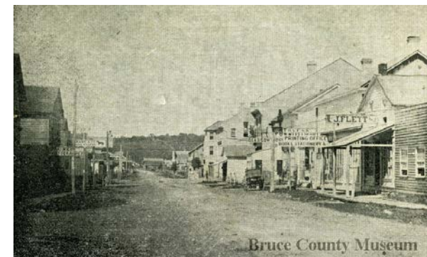
Durham Street, looking west from Post Office, 1872
