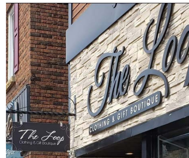
Stone veneer facade
