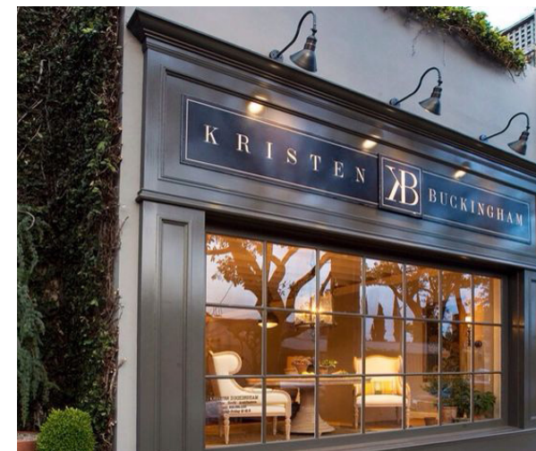
Multiple 'gooseneck' lights in a row will illuminate sign.
