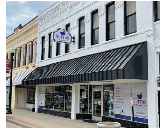
Permanent aluminum awning
