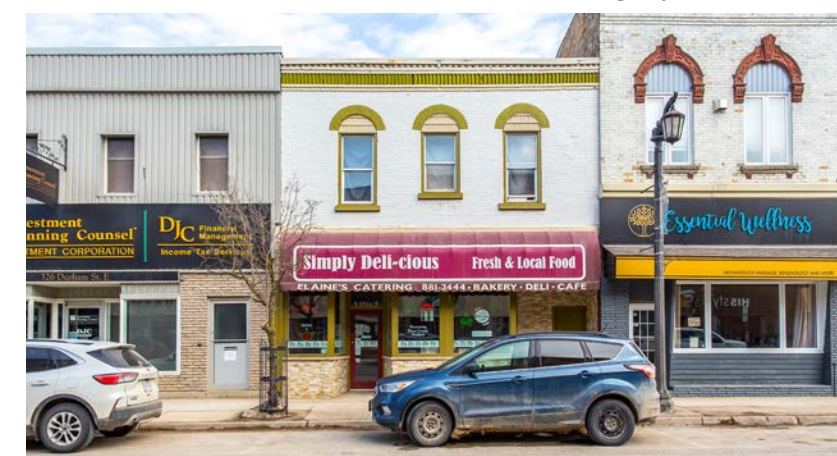
Existing Façade, March 2023
