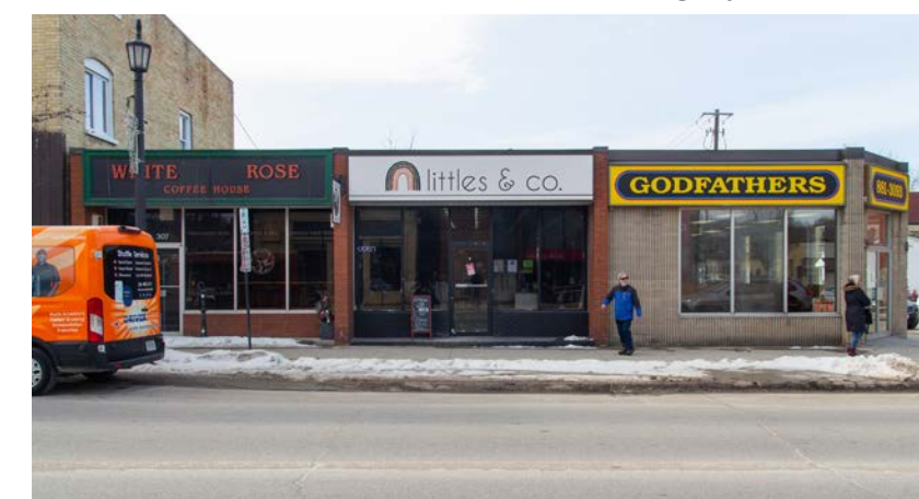
Existing Façade, March 2023
