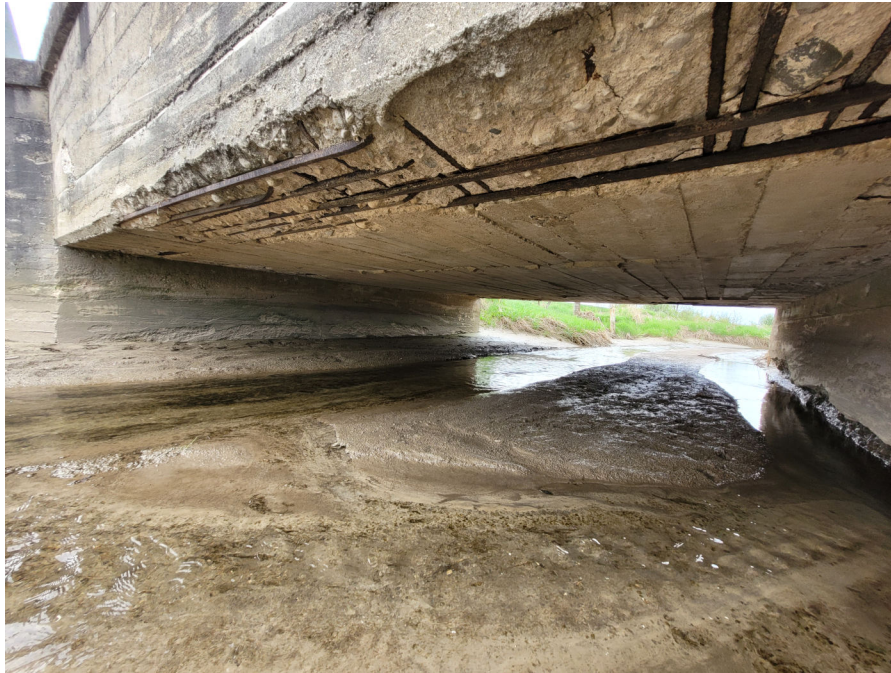
View of abutment wall and soffit, typical.
