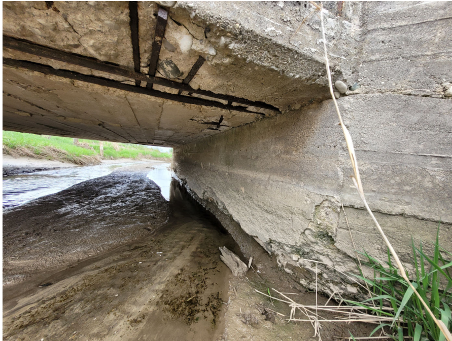
View of abutment wall and soffit, typical.
