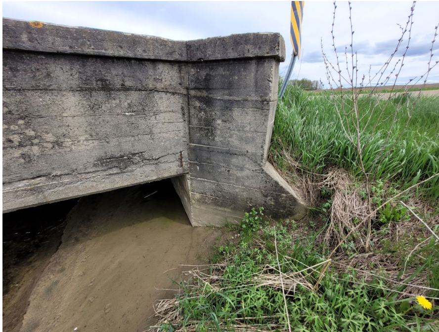
View of wingwall, typical.
