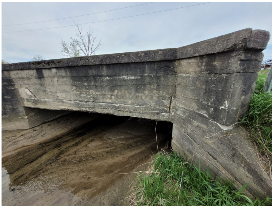
View of exterior of parapet wall, typical.
