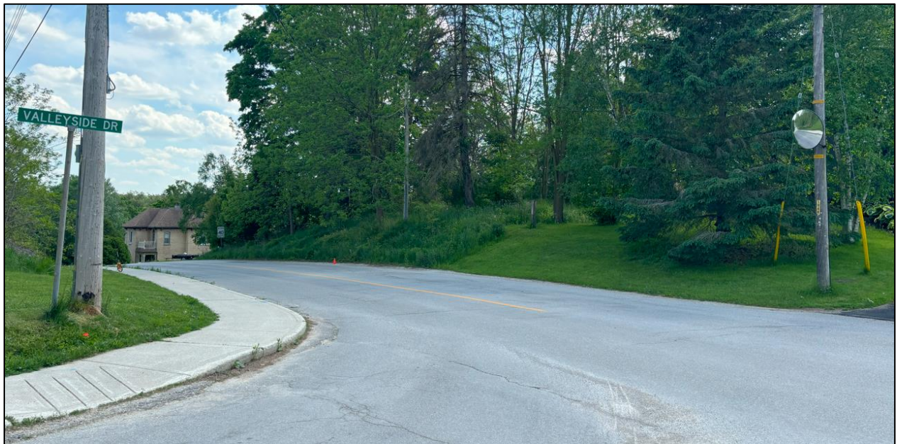
Figure 13: View of a motorist looking left from Valleyside Drive – Departure sight distance (TNS, 2024).
