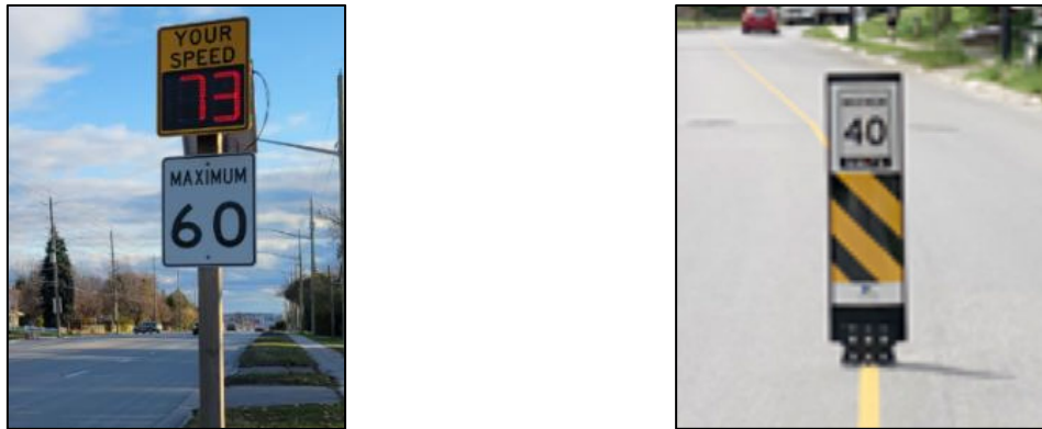
Figure 15: Radar speed sign (shown left); centreline bollard (shown right).
