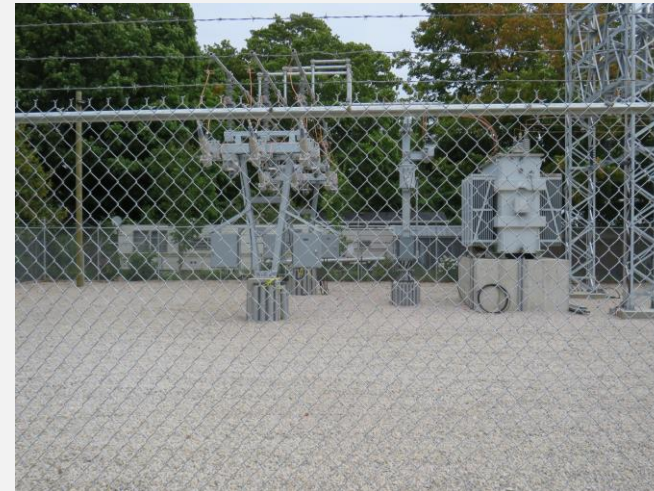
Teeswater Under Construction 2024
