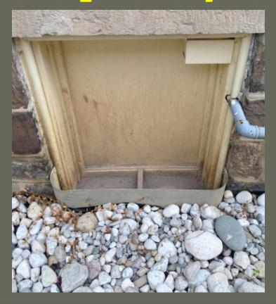
Apart from security concerns, rainwater was running into the basement, causing dampness, odour and the potential for mould.
