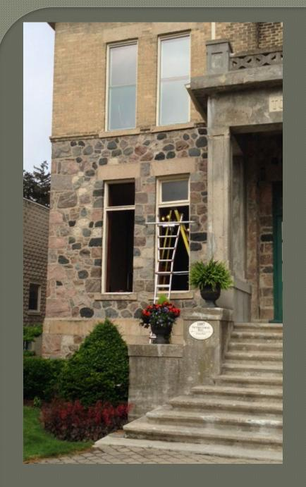
This involved removal and refurbishment of the old windows, and installation of insulated glass on the outside of the old windows, protecting them from further deterioration.
