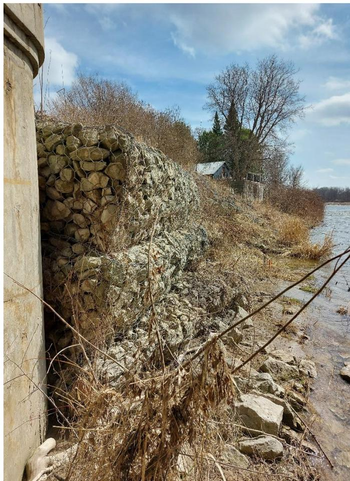
Gabion basket erosion protection
