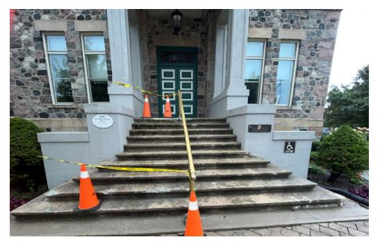
The new steps will be in the exact same location and configuration as the old steps, and the centre brass railing will be removed, and replaced in the same location on the new porch.
