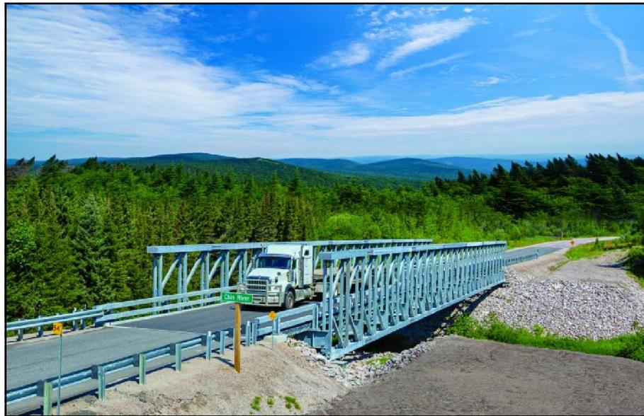
**Photo P-4** - Structural Steel Panel Bridge (Algonquin Bridge).
