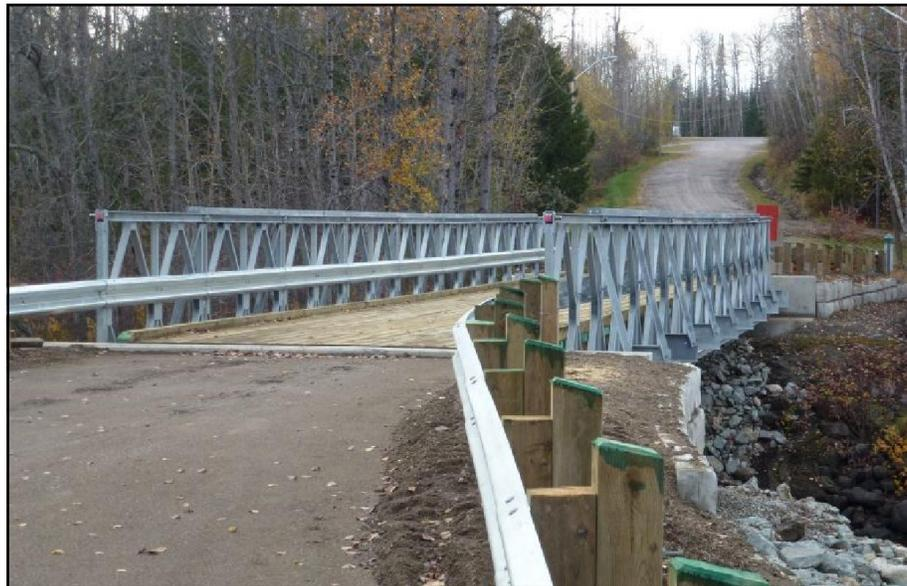
**Photo P-2** - Bailey Style Steel Panel Bridge (Algonquin Bridge).
