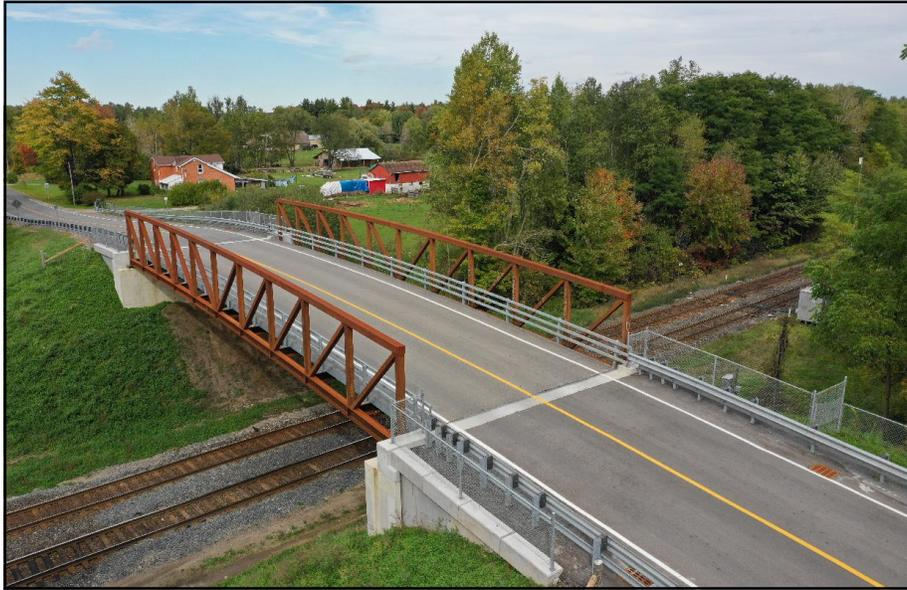
**Photo P-5** - Structural Steel Panel Bridge (Iron Bridge).
