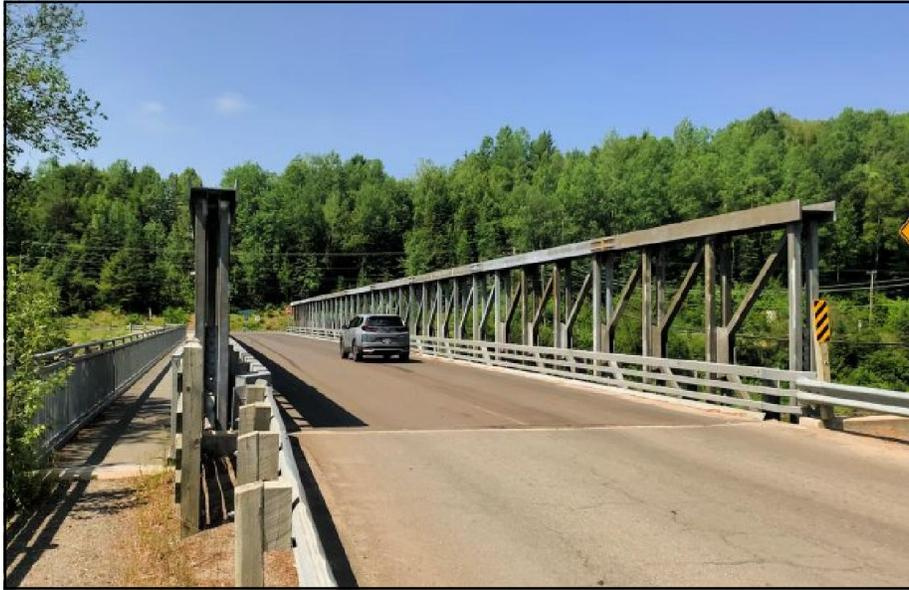
**Photo P-3** - Structural Steel Panel Bridge (Algonquin Bridge).
