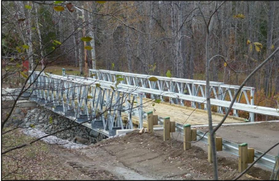
**Photo P-1** - Bailey Style Steel Panel Bridge (Algonquin Bridge).
